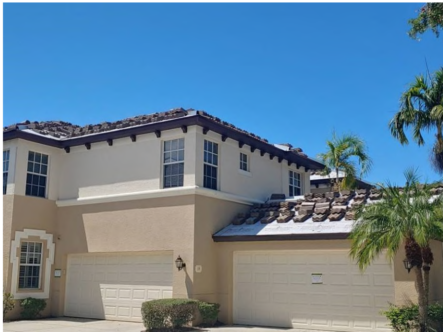
Photograph #14: Roof tiles were set into place for installation on building 21740.
