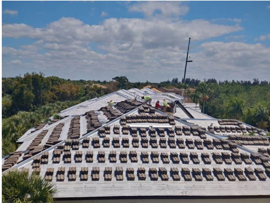
Photograph #13: Roof tiles were set into place for installation on building 21731.
