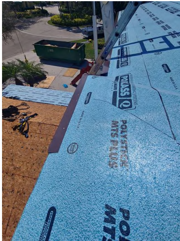
Photograph #9: Drip edge installation was in progress on building 7861.
