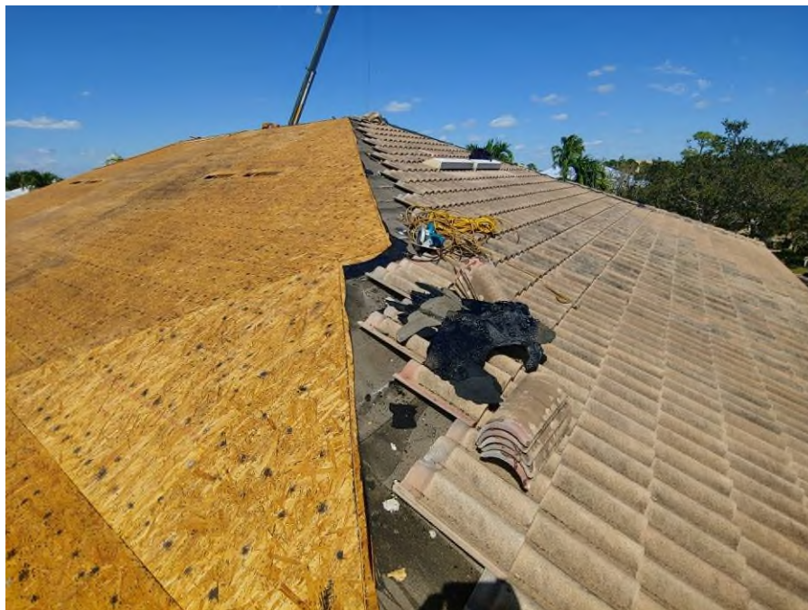
Photograph #10: Roof tile removal was in progress on building 21740.
