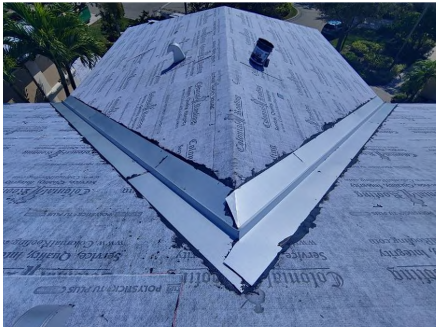
Photograph #2: V-crimp metal valley flashing installation was in progress on building 7851.
