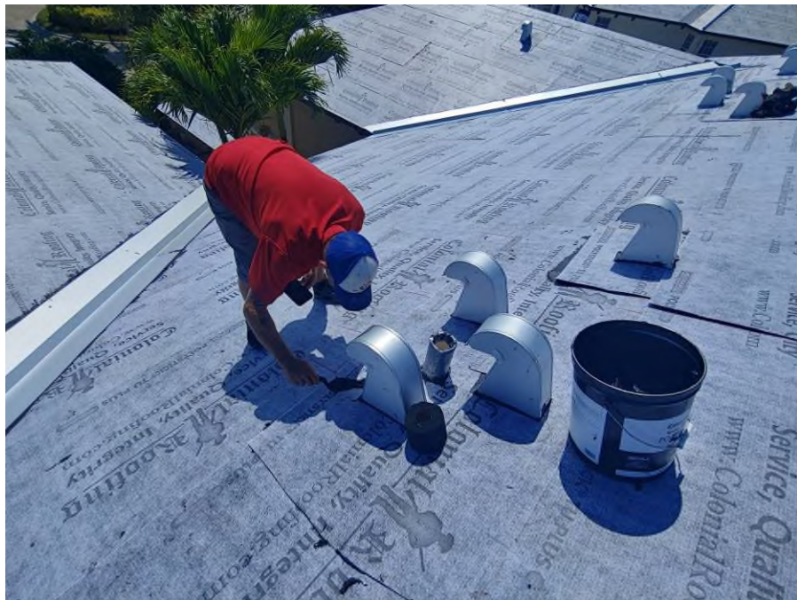
Photograph #4: Exhaust vent installation was in progress on building 7851.
