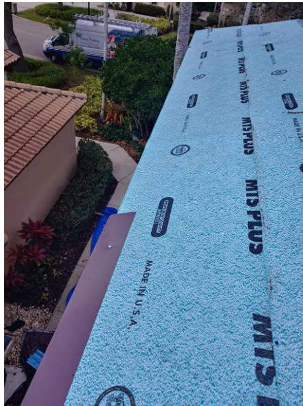
Photograph #5: Drip edge installation was in progress on building 7870.
