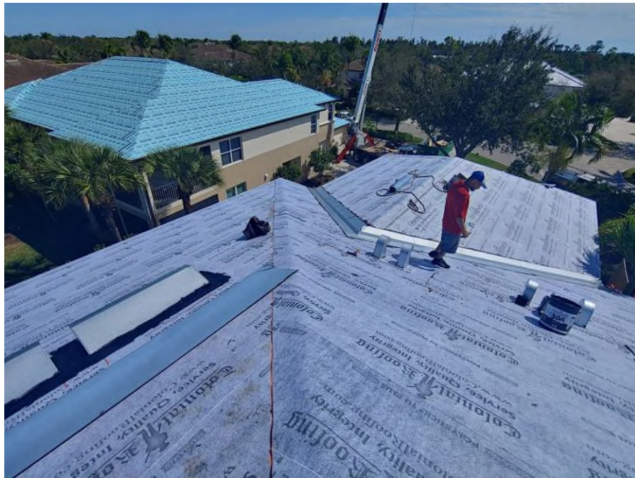
Photograph #3: Exhaust vent installation was in progress on building 7851.
