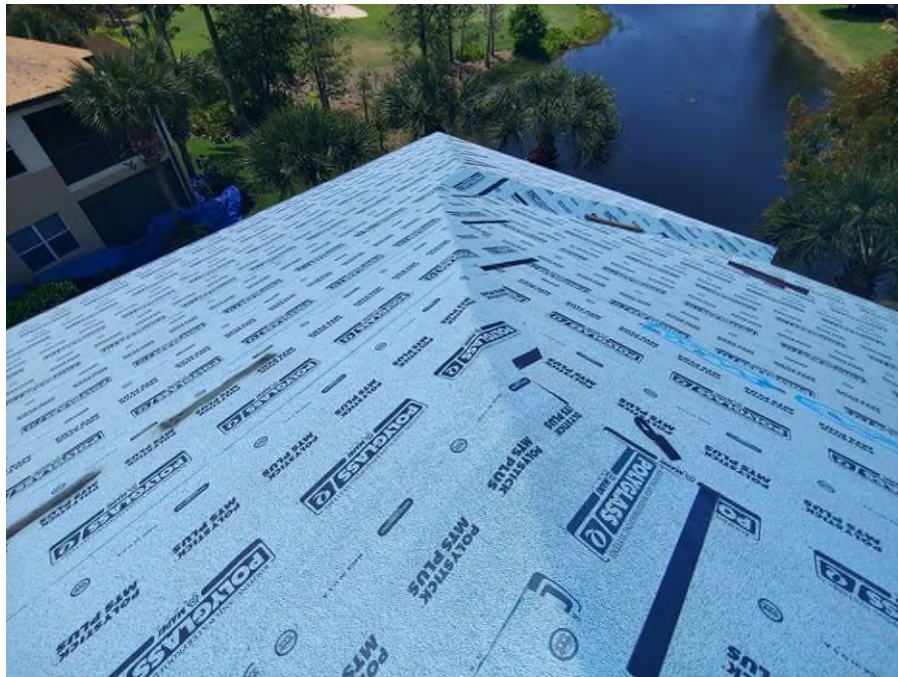
Photograph #21: Polystick MTS Plus underlayment was completed on building 21810.
