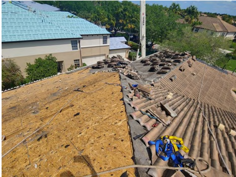
Photograph #25: Roof tile removal was in progress on building 21820.
