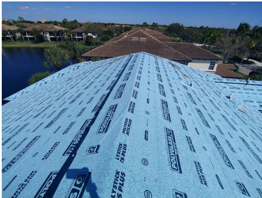
Photograph #8: Polystick MTS Plus underlayment installation was in progress on building 7861.
