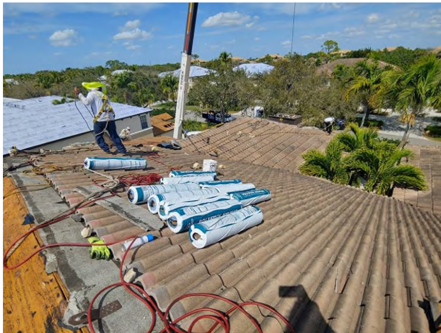
Photograph #10: Observed work-in-progress was completed on building 21750.
