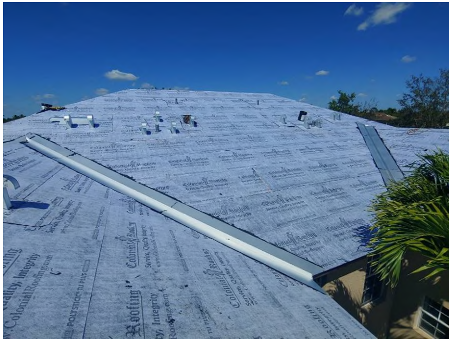
Photograph #1: Second layer of underlayment installation was completed on building 7851.
