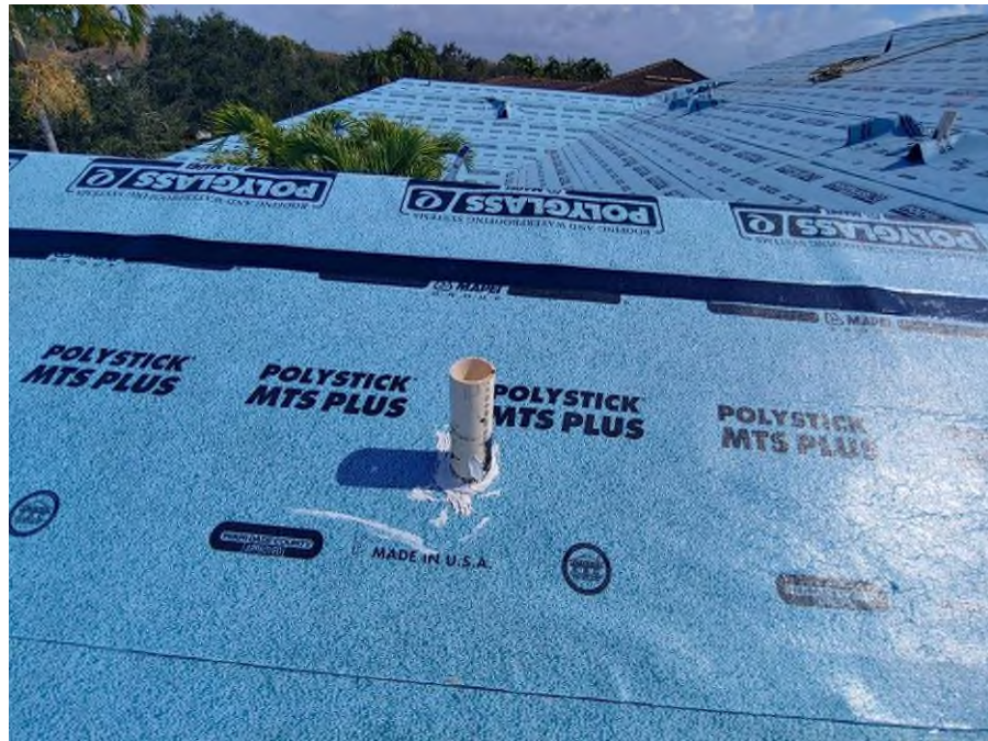
Photograph #9: Sealant application on Vent-pipe was in progress on building 21720.
