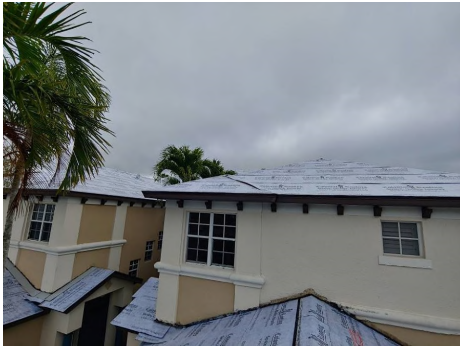
Photograph #5: Second layer of underlayment installation was in progress on building 7860.
