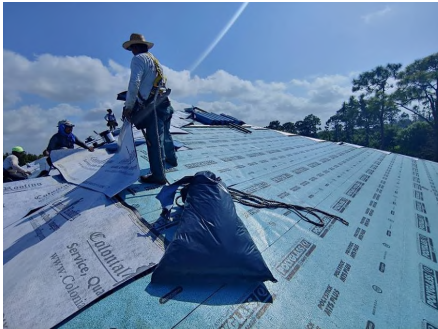
Photograph #11: Polystick MTS Plus underlayment installation was completed on building 7850.
