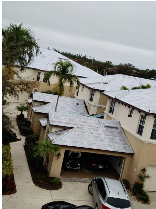
Photograph #10: Second layer of underlayment installation was in progress on building 21710.
