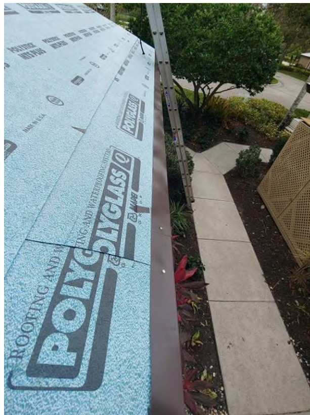
Photograph #18: Drip-edge flashing installation was in progress on building 21721.
