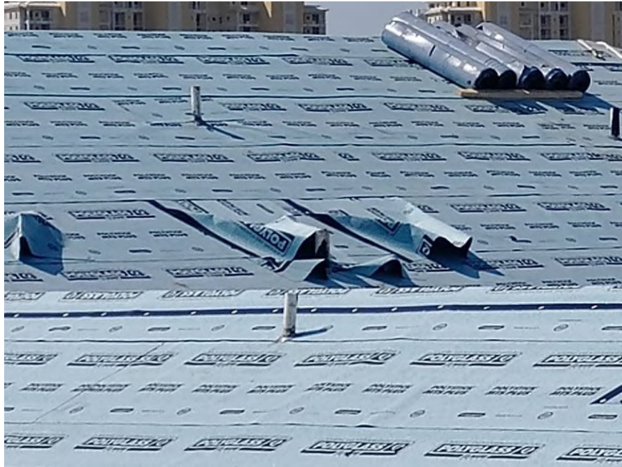
Photograph #7: Polystick MTS Plus underlayment installation was completed on building 21710.
