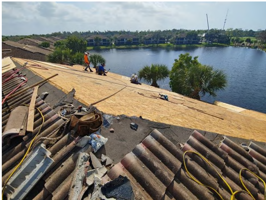
Photograph #16: Roof tile removal was in progress on building 21720.
