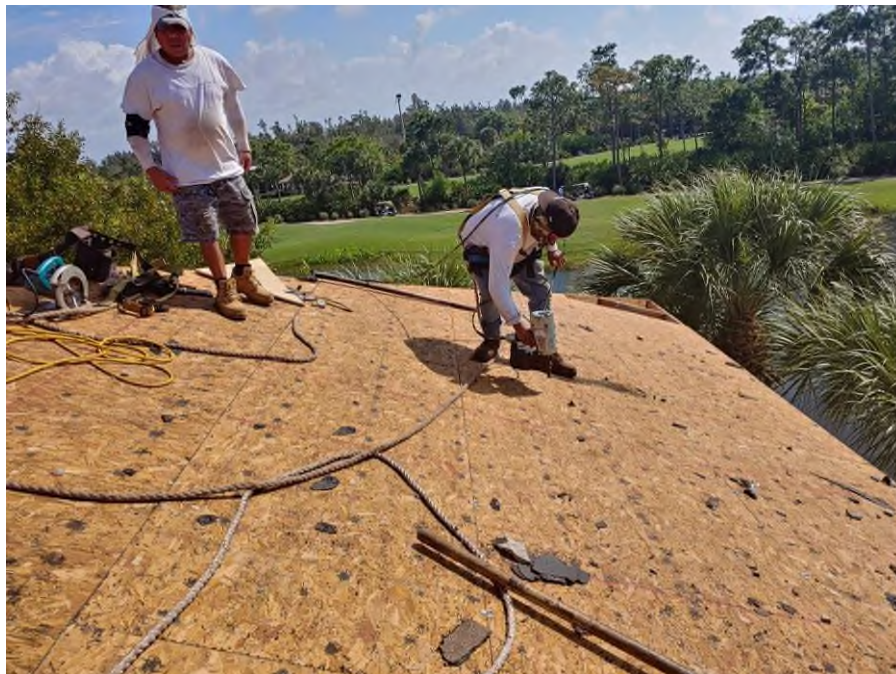
Photograph #4: Re-nail pattern at plywood sheathing was in progress on building 7860.
