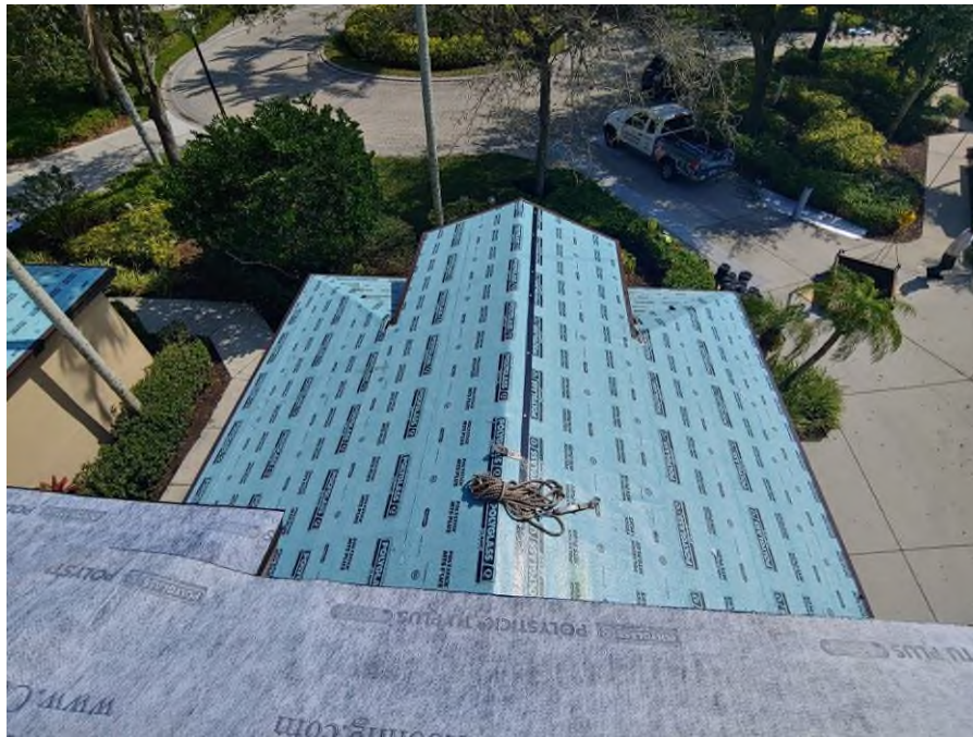
Photograph #7: Polystick MTS Plus underlayment installation was completed on building 7841.
