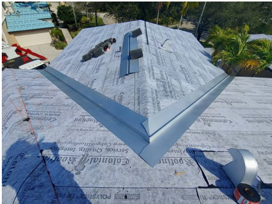
Photograph 4: V-crimp metal Valley flashing installation was in progress on building 7840.
