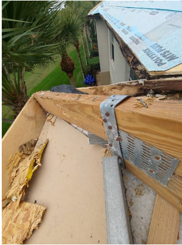
Photograph #21: Existing strap clips on trusses have the required minimum quantity of nails on building 21731. Installation of new hurricane truss anchor straps (HGAM10) is not required.
