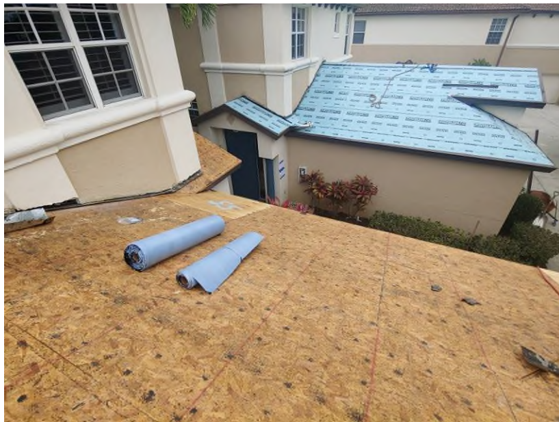
Photograph #2: Polystick MTS Plus underlayment installation was in progress on building 7851.
