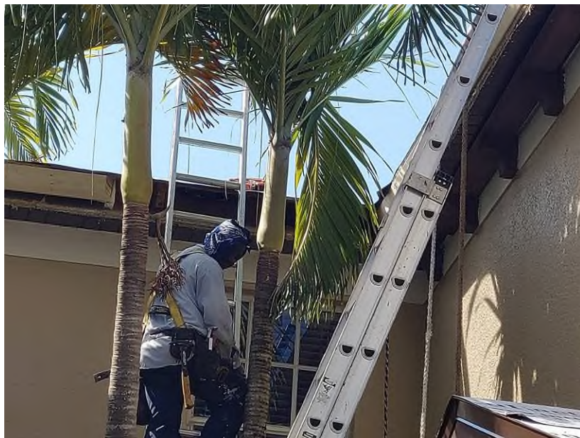
Photograph #14: Fascia repair was in progress on building 21710.
