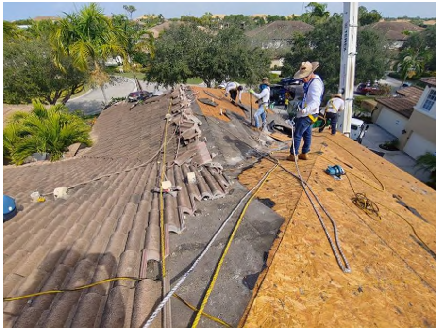
Photograph #17: Roof tile removal was in progress on building 21720.
