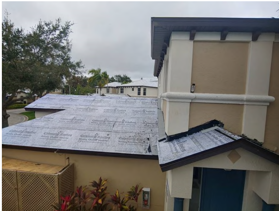
Photograph #17: Second layer of underlayment installation was in progress on building 21721.
