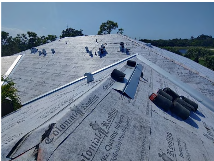
Photograph #2: Exhaust vent installations were in progress on building 7840.
