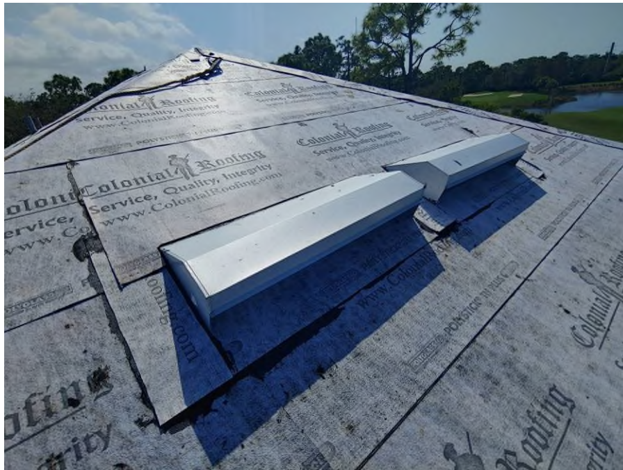
Photograph #3: Exhaust vent installations were in progress on building 7840.
