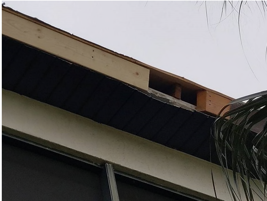
Photograph #19: Fascia repair was in progress on building 21721.
