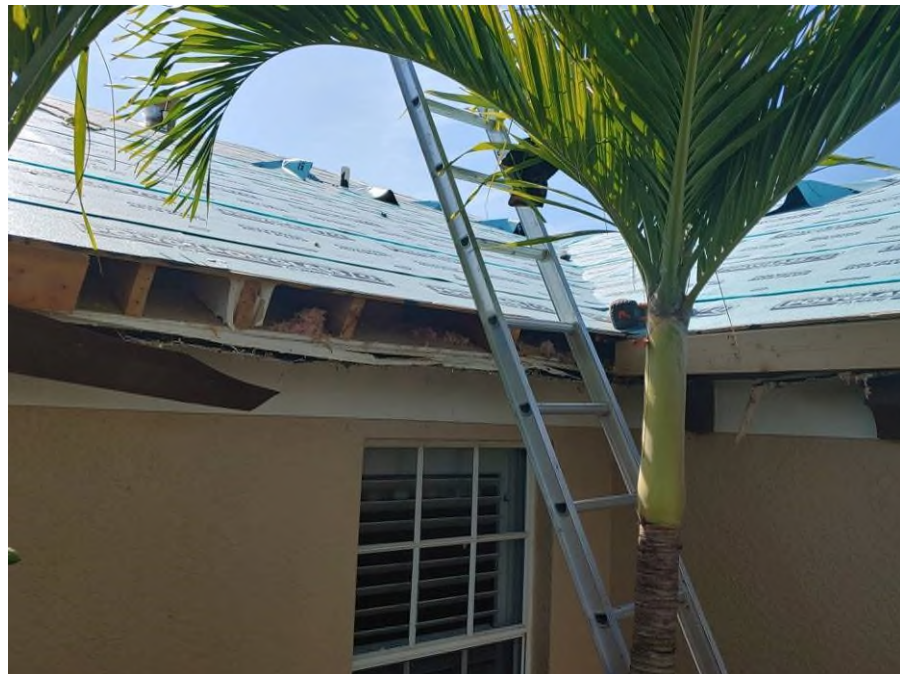
Photograph #10: Fascia repair was in progress on building 21720.
