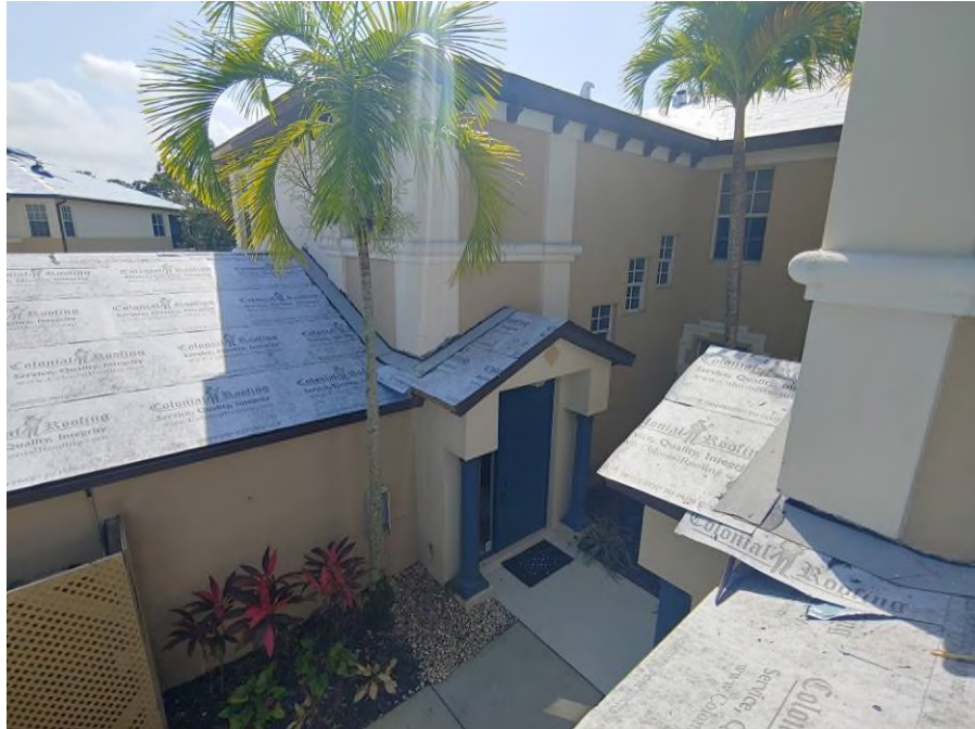
Photograph #1: Second layer of underlayment installation was completed on building 7840.
