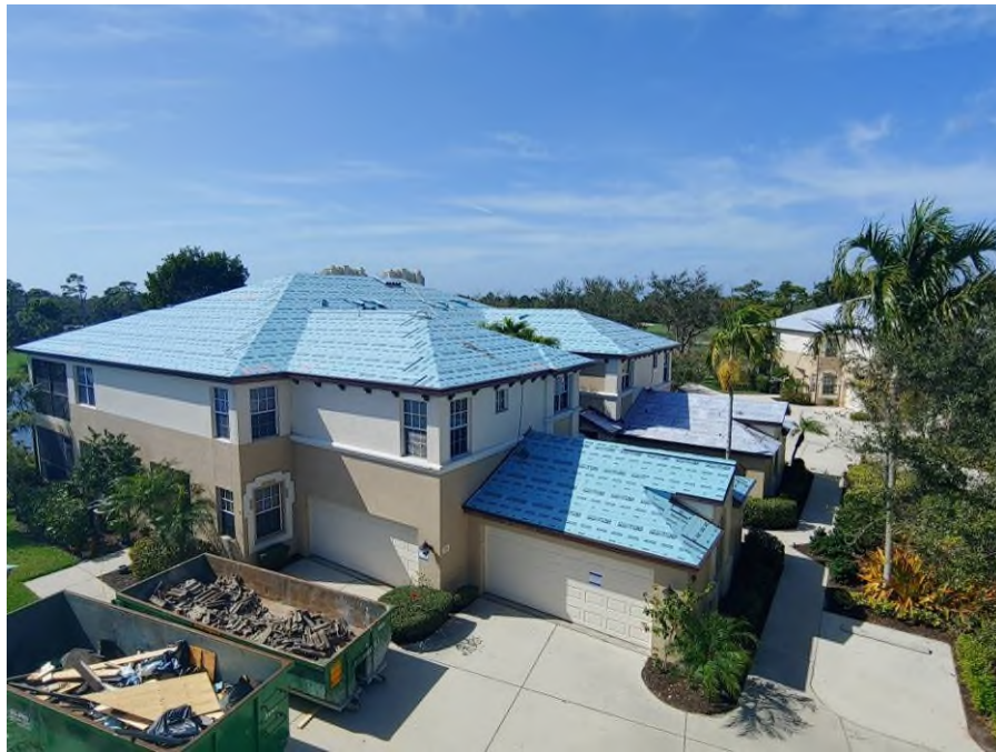
Photograph #5: Polystick MTS Plus underlayment installation was completed on building 21710.
