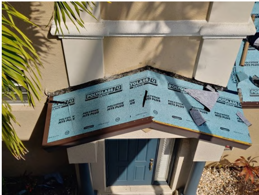
Photograph #8: Drip-edge flashing installation was in progress on building 7841.
