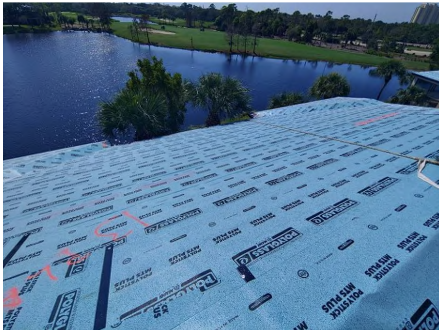
Photograph #8: Polystick MTS Plus underlayment installation was completed on building 21720.
