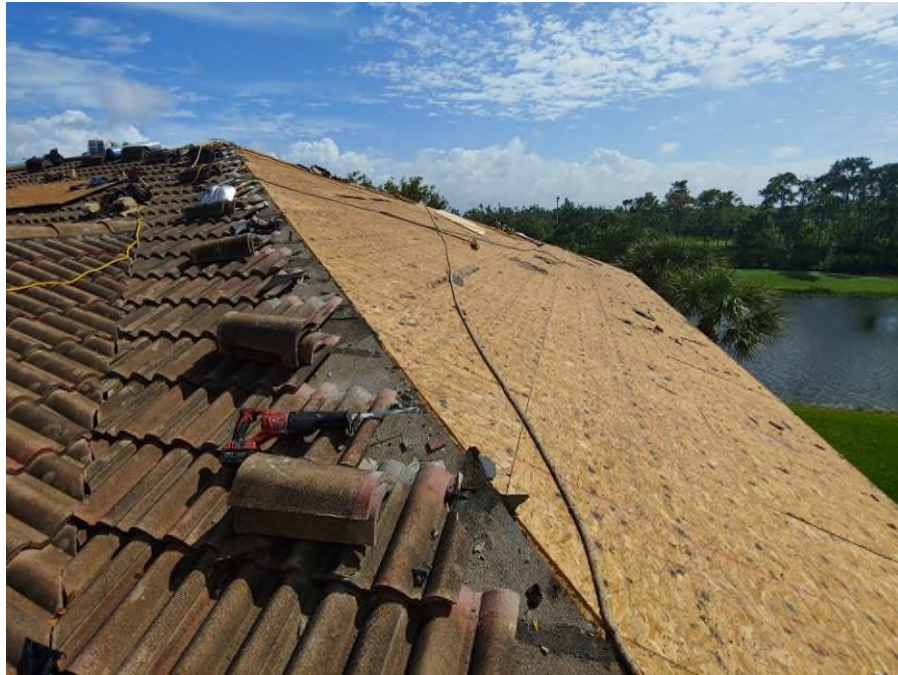
Photograph #1: Roof tile removal was in progress on building 7860.
