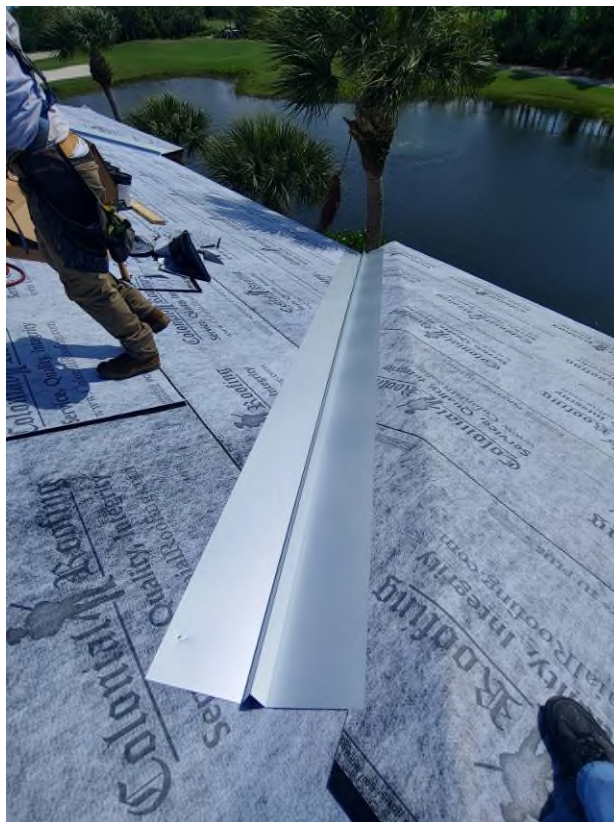
Photograph #12: V-crimp metal Valley flashing installation was in progress on building 7850.
