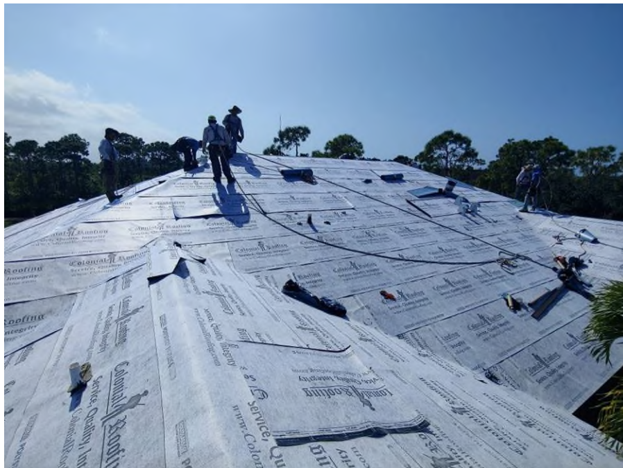
Photograph #10: Second layer of underlayment installation was in progress on building 7850.
