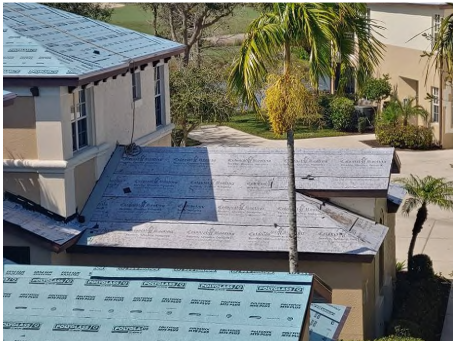
Photograph #6: Second layer of underlayment installation was in progress on building 21710.
