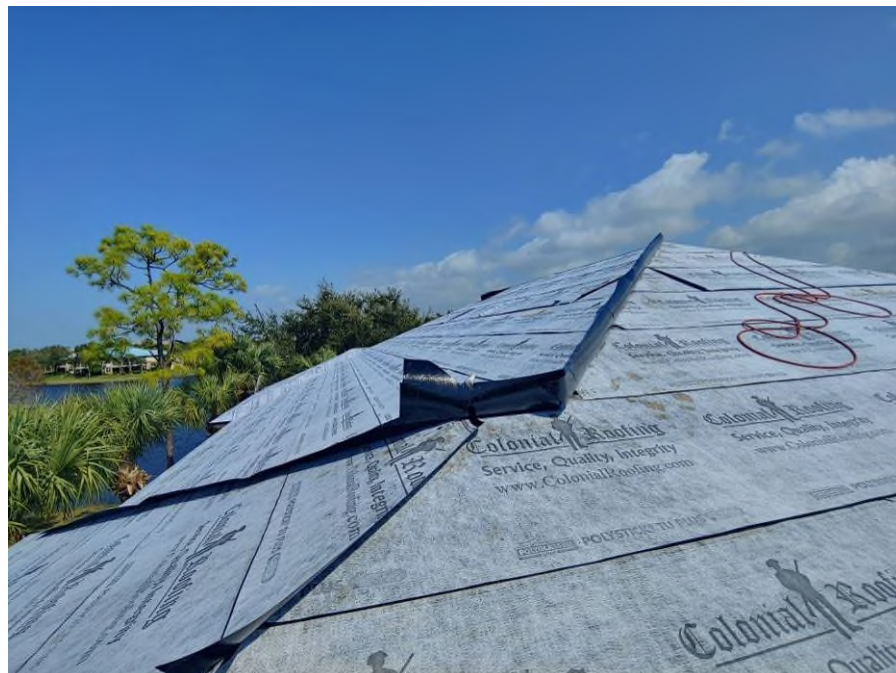
Photograph #6: Second layer of underlayment installation was in progress on building 7841.
