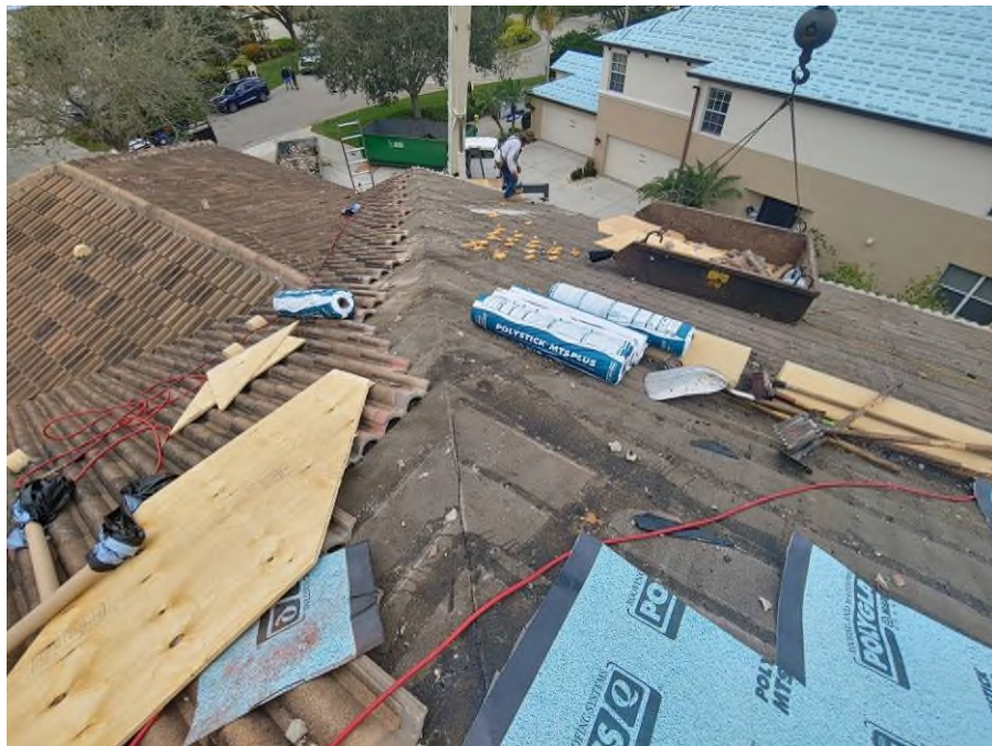
Photograph #20: Roof tile removal was in progress on building 21731.
