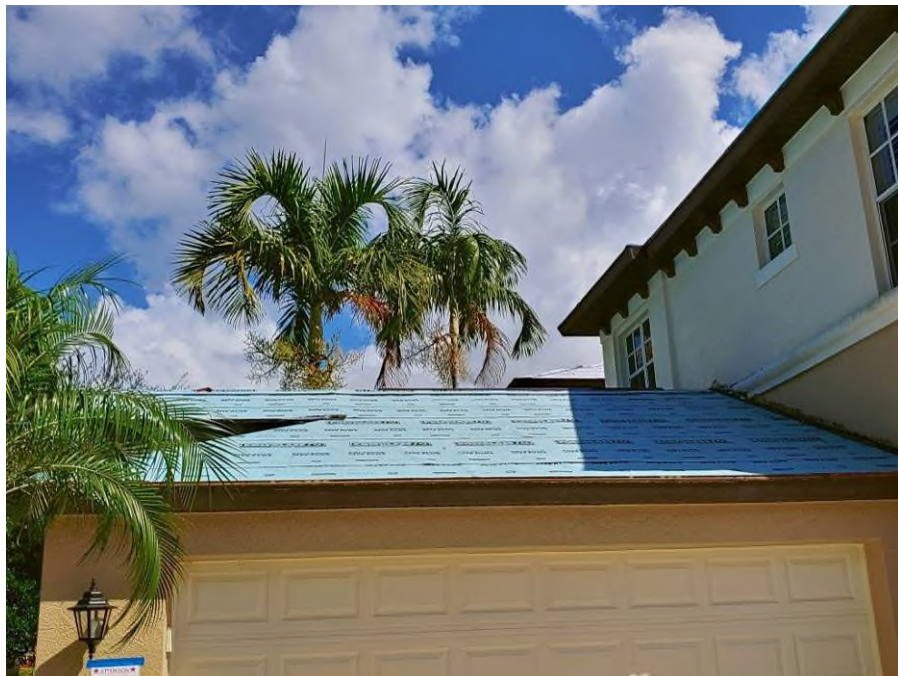
Photograph #10: Polystick MTS Plus underlayment installation was completed on building 7860.
