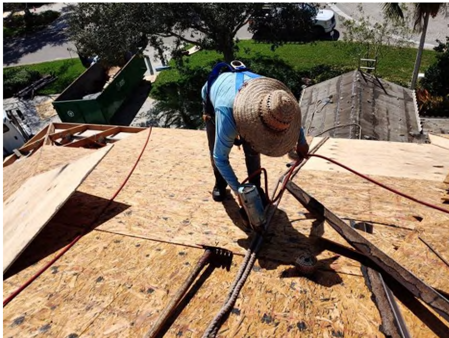
Photograph #6: Re-nail pattern at plywood sheathing was in progress on building 21721.
