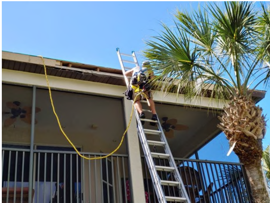
Photograph #5: Fascia repair was in progress on building 21721.
