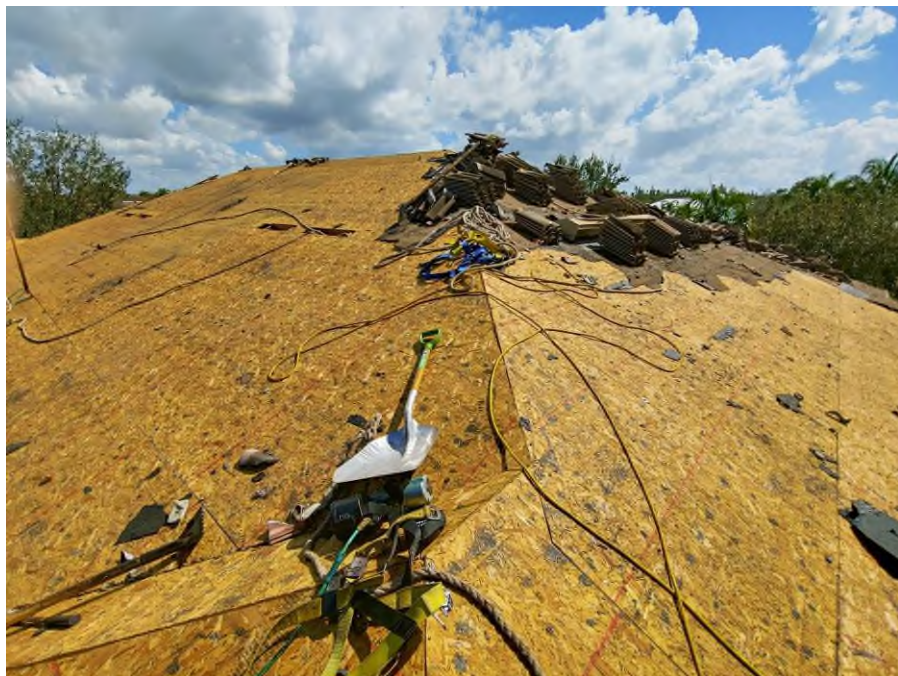
Photograph #2: Roof tile removal was in progress on building 7851.
