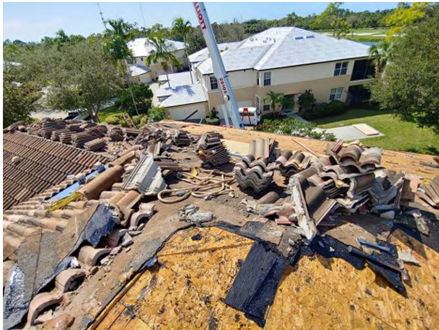
Photograph #1: Roof tile removal was in progress on building 7851.
