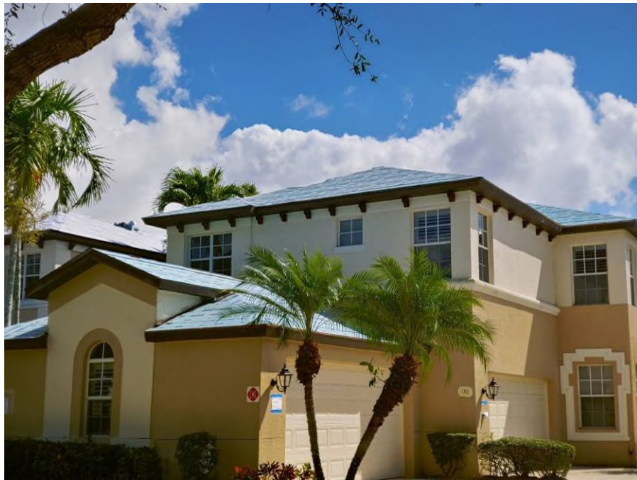
Photograph #9: Second layer of underlayment installation was in progress on building 7860.
