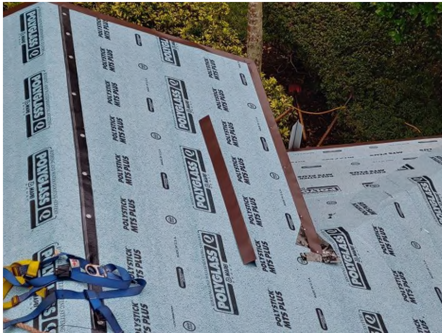
Photograph #3: Drip-edge flashing installation was in progress on building 7851.
