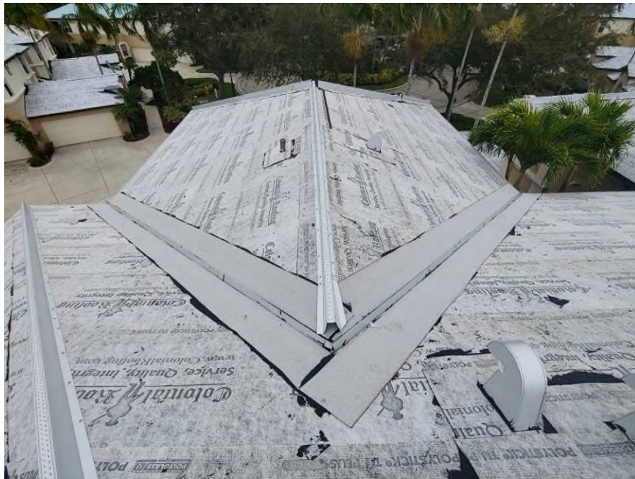
Photograph #7: V-crimp metal valley flashing, and hip/ridge metal channel installations were in progress on building 21700.
