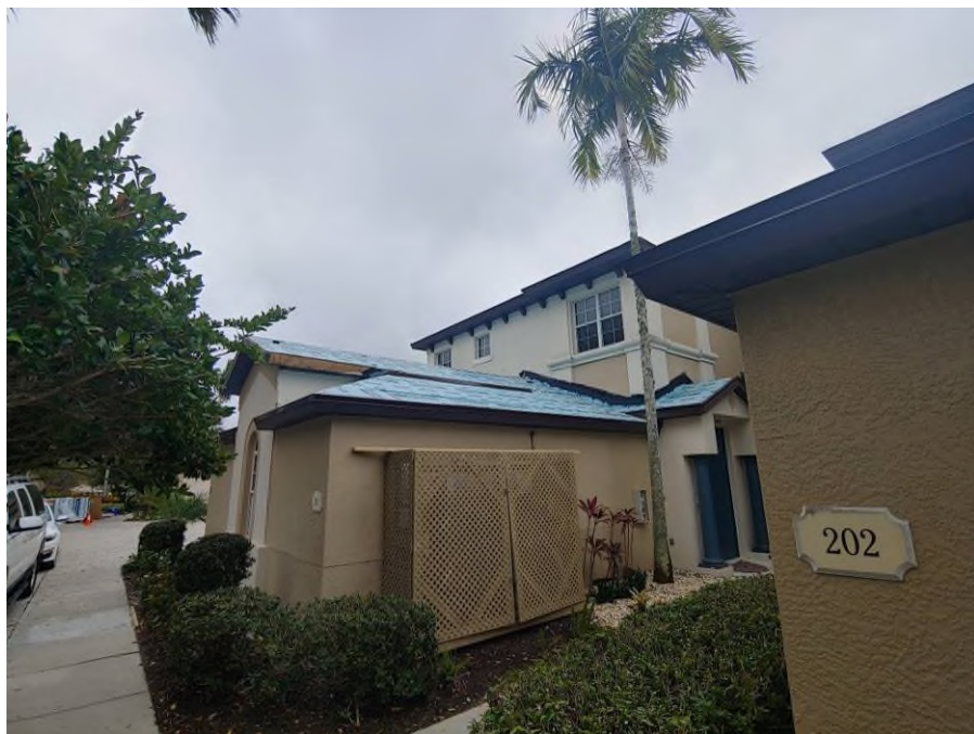
Photograph #14: Second layer of underlayment installation was in progress on building 21720.
