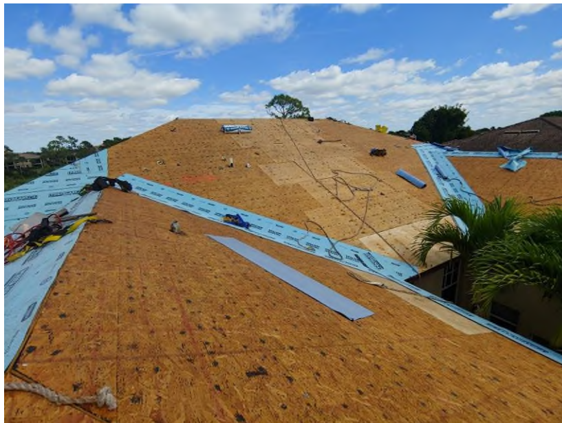
Photograph #8: Polystick MTS Plus underlayment installation was in progress on building 21731.
