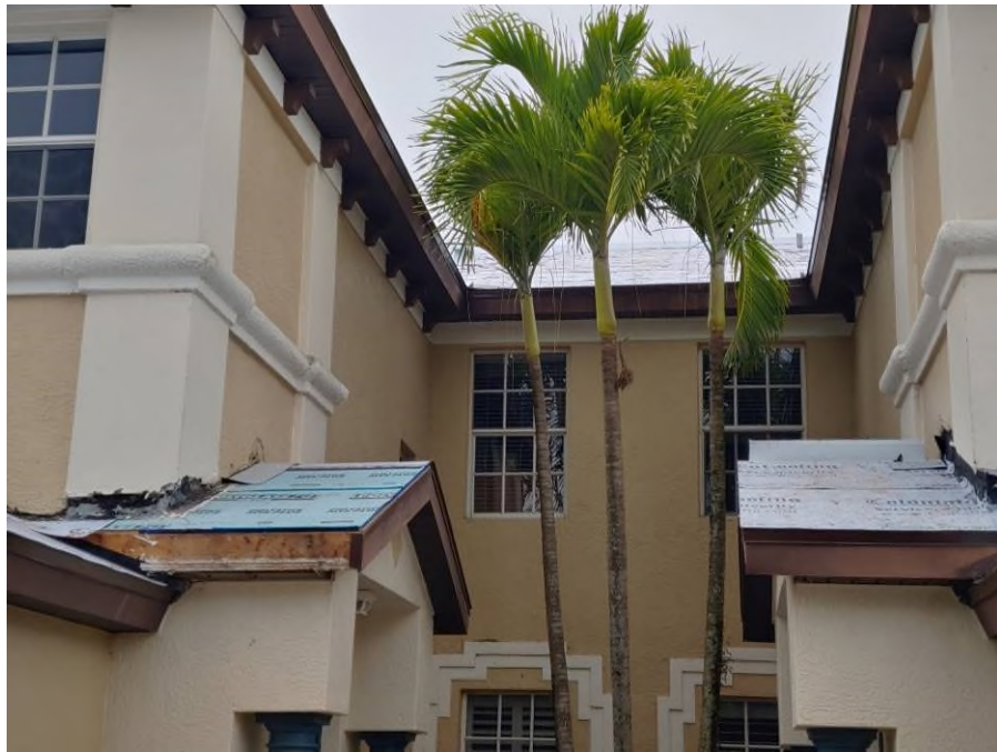
Photograph #11: Fascia repair was in progress on building 21710.
