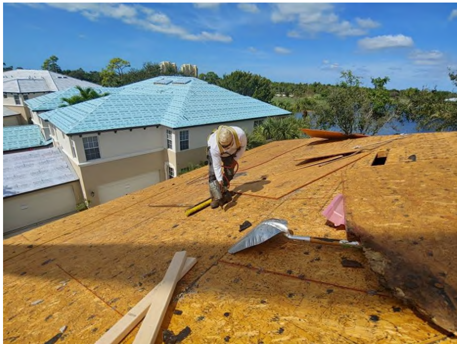
Photograph #4: Re-nail pattern at plywood sheathing was in progress on building 7861.
