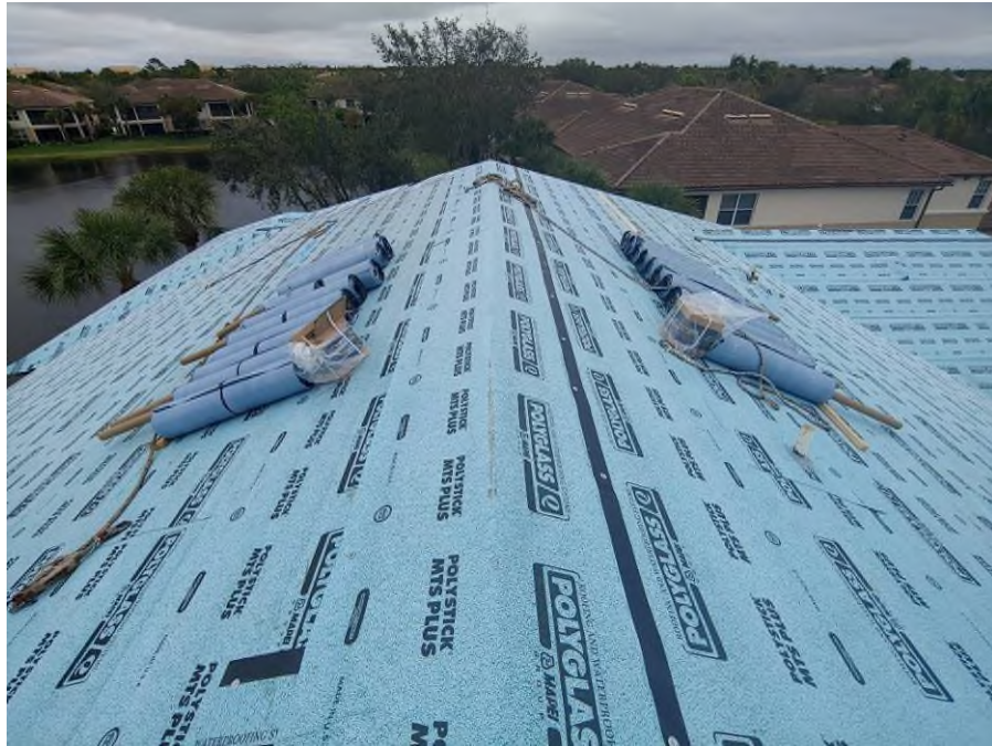
Photograph #1: Polystick MTS Plus underlayment installation was in progress on building 7851.
