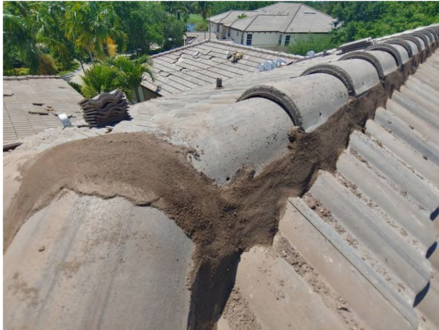
Photograph #9: Mortar adhesive application was in progress on building 21711.
