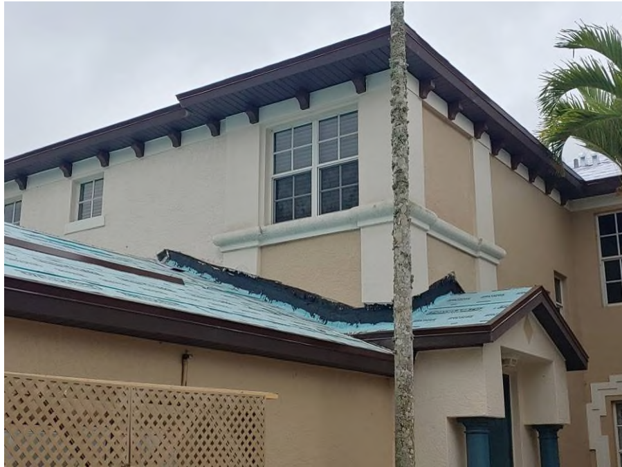
Photograph #15: Drip-edge flashing installation was in progress on building 21720.
