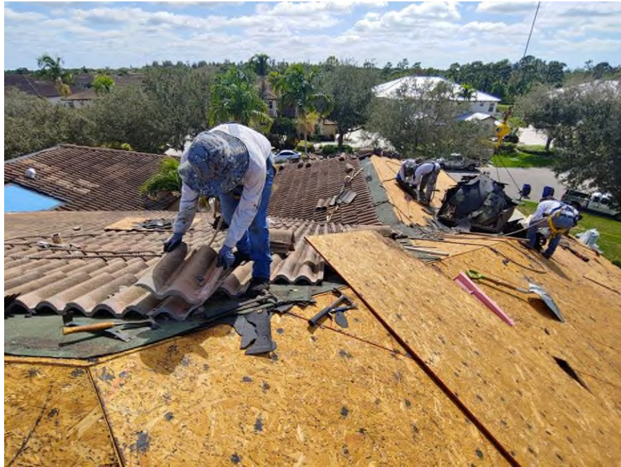
Photograph #1: Roof tile removal was in progress on building 7861.
