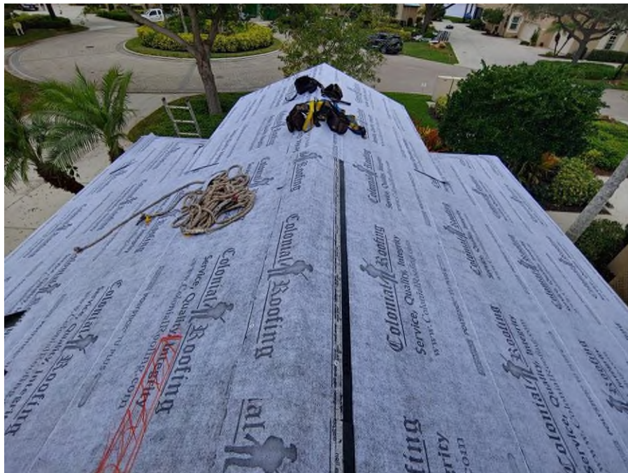
Photograph #4: Second layer of underlayment installation was in progress on building 7860.
