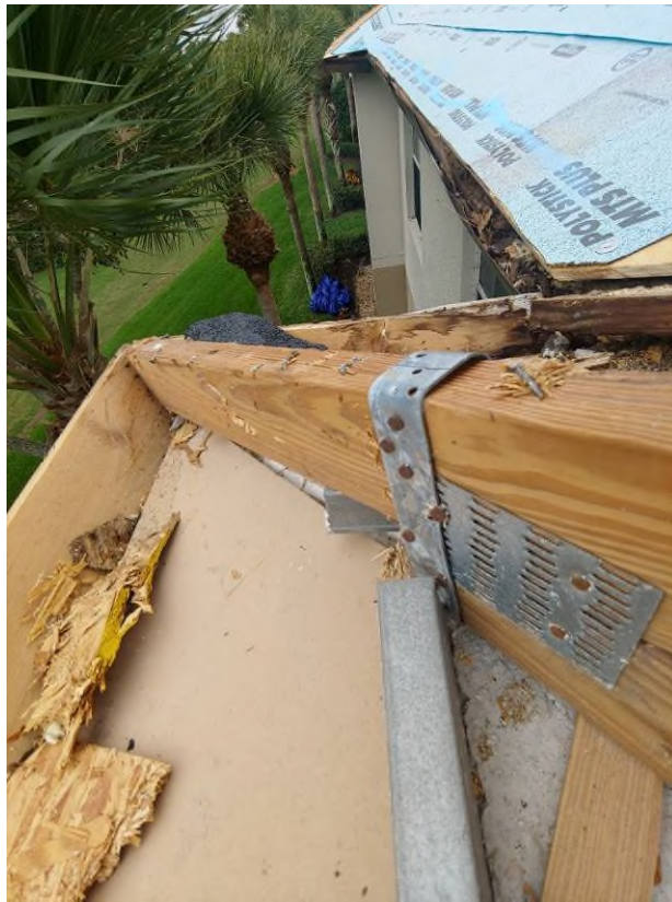
Photograph #21: Existing strap clips on trusses have the required minimum quantity of nails on building 21731. Installation of new hurricane truss anchor straps (HGAM10) is not required.
