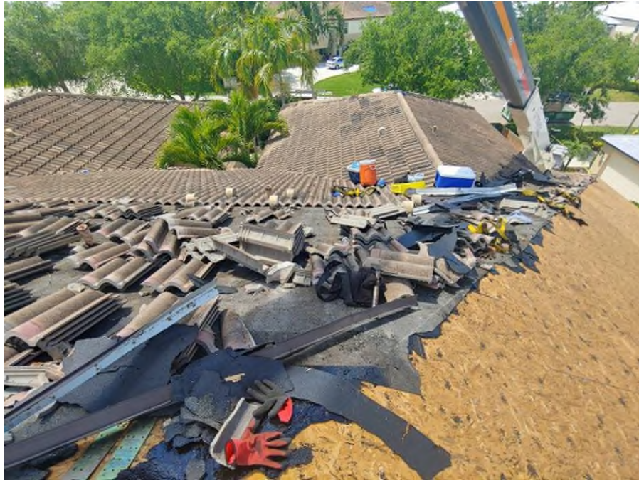
Photograph #15: Roof tile removal was in progress on building 21781.
