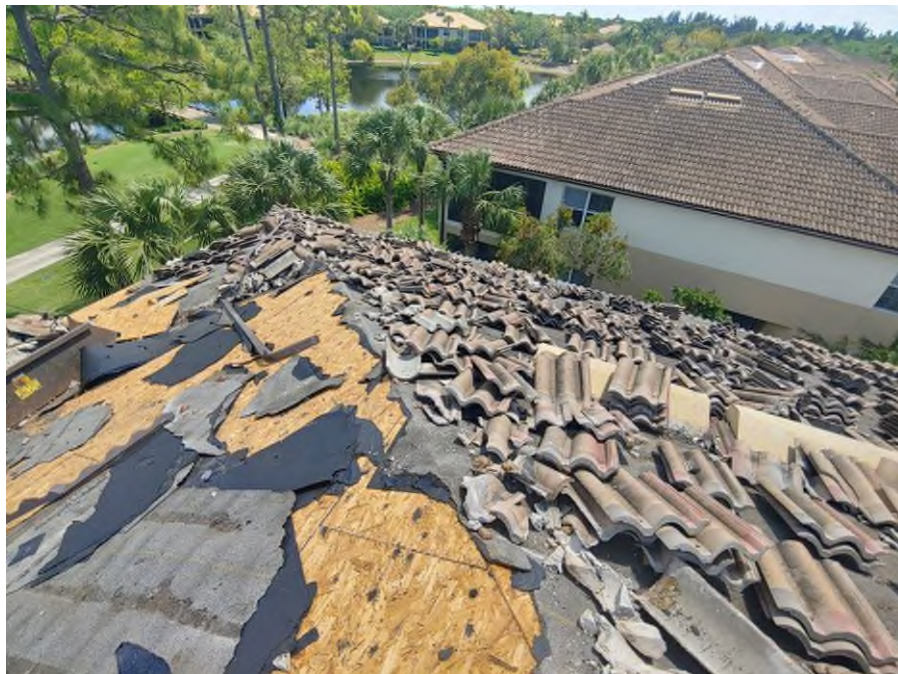
Photograph #16: Roof tile removal was in progress on building 21781.
