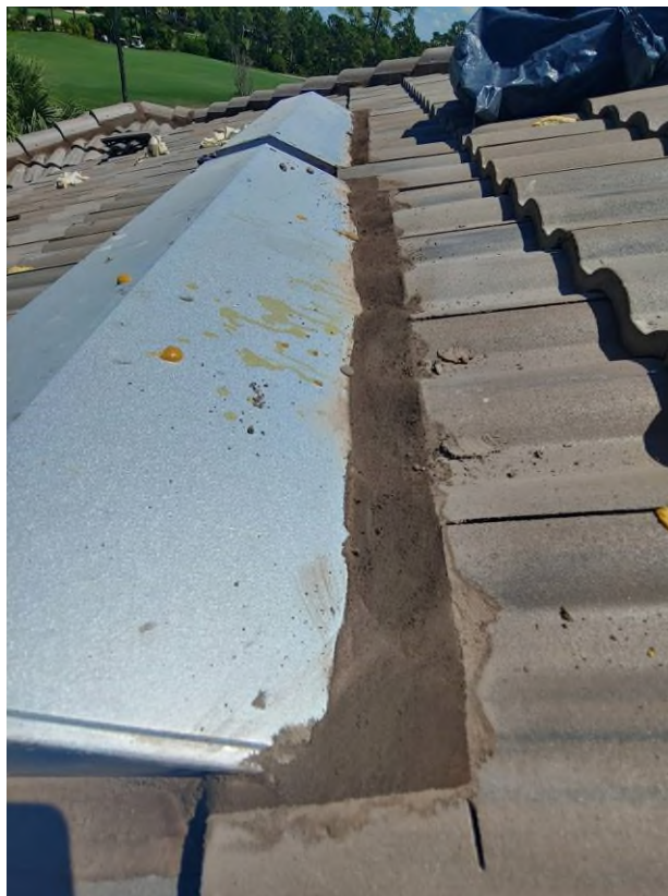
Photograph #8: Mortar adhesive application was in progress on building 21711.
