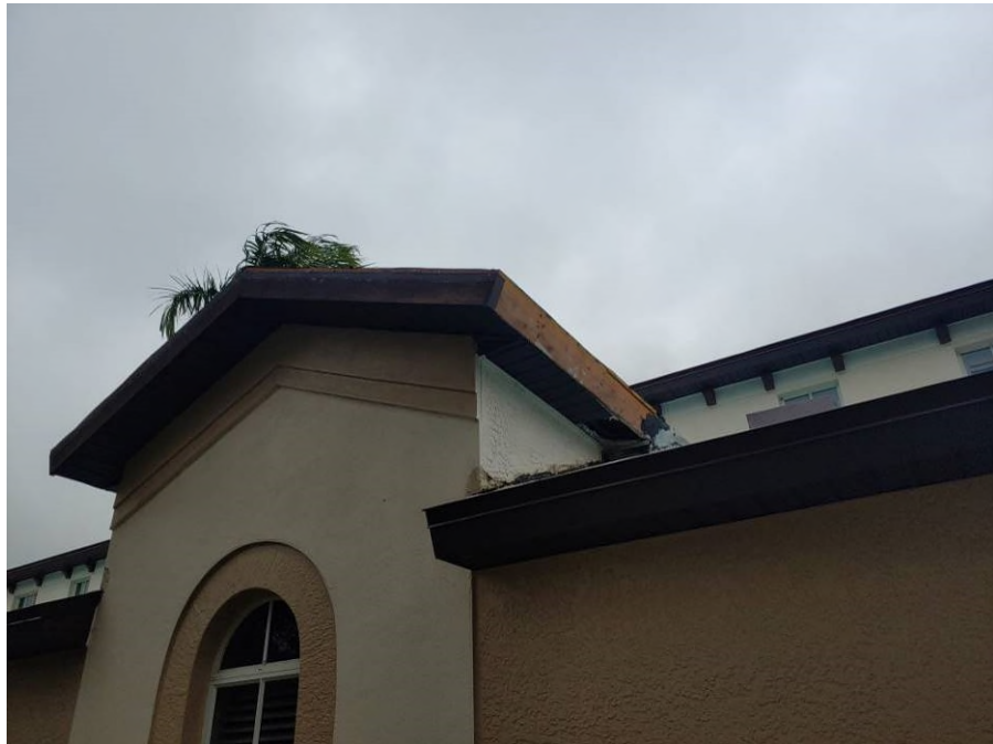
Photograph #16: Fascia repair was in progress on building 21720.
