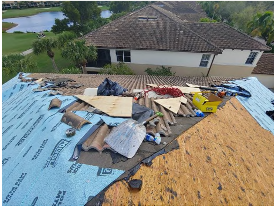
Photograph #7: Roof tile removal was in progress on building 21731.
