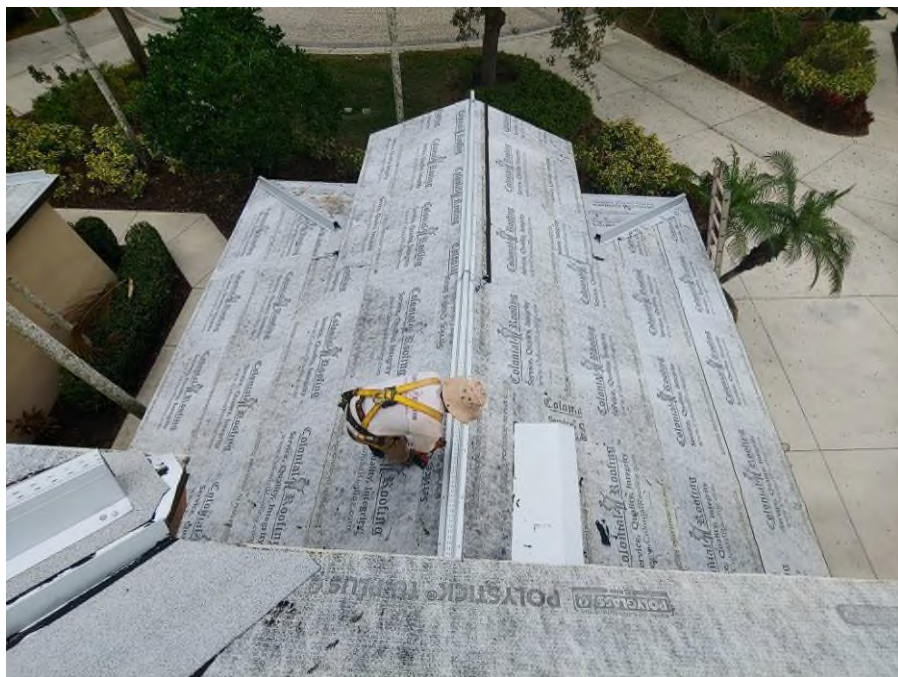
Photograph #8: V-crimp metal valley flashing, and hip/ridge metal channel installations were in progress on building 21700.
