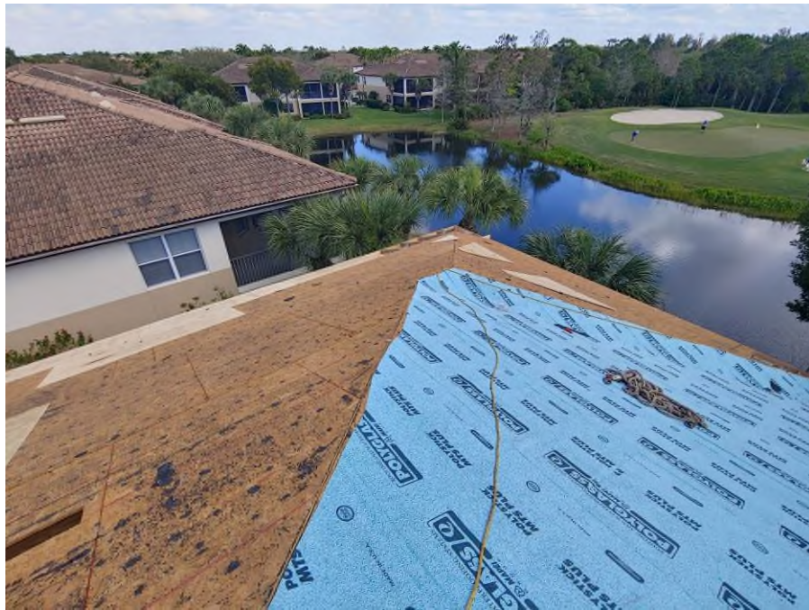
Photograph #3: Polystick MTS Plus underlayment installation was in progress on building 7870.
