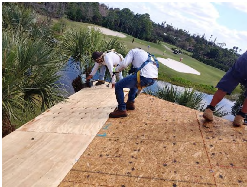
Photograph #4: Re-nail pattern at the plywood sheathing was in progress on buildings 7870.
