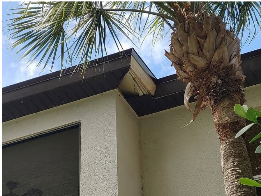
Photograph #6: Fascia repair was in progress on building 7870.
