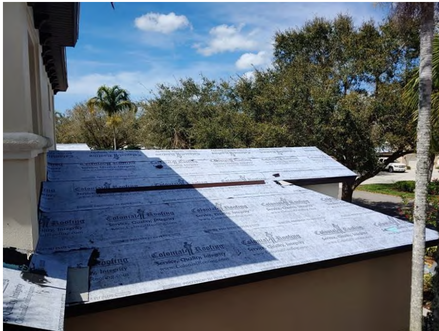
Photograph #9: Second layer of underlayment was in progress on building 21740.
