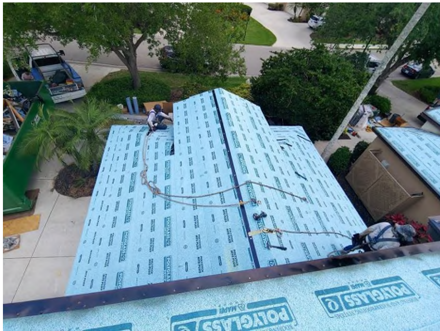
Photograph #6: Drip-edge flashing installation was in progress on building 21840.
