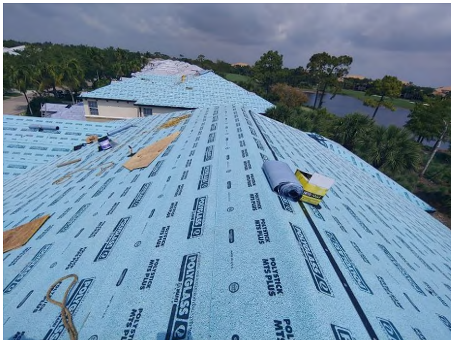
Photograph #12: Polystick MTS Plus underlayment installation was in progress on building 21801.
