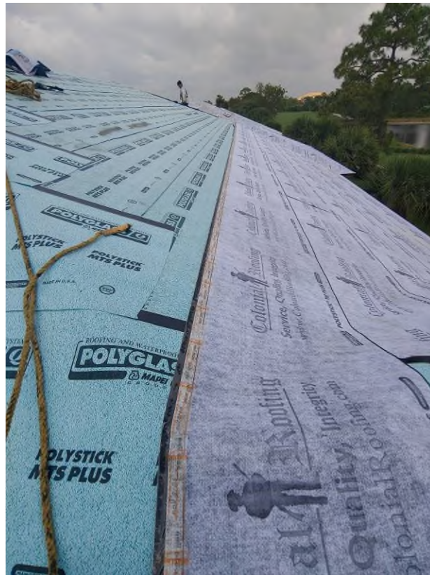
Photograph #3: Second layer of underlayment installation was in progress on building 21791.
