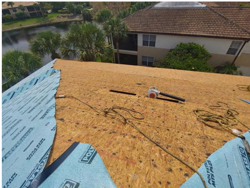
Photograph #8: Roof tile removal was completed on building 21801.
