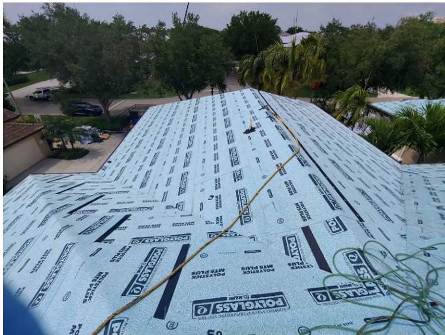
Photograph #2: Polystick MTS Plus underlayment installation was completed on building 21791.
