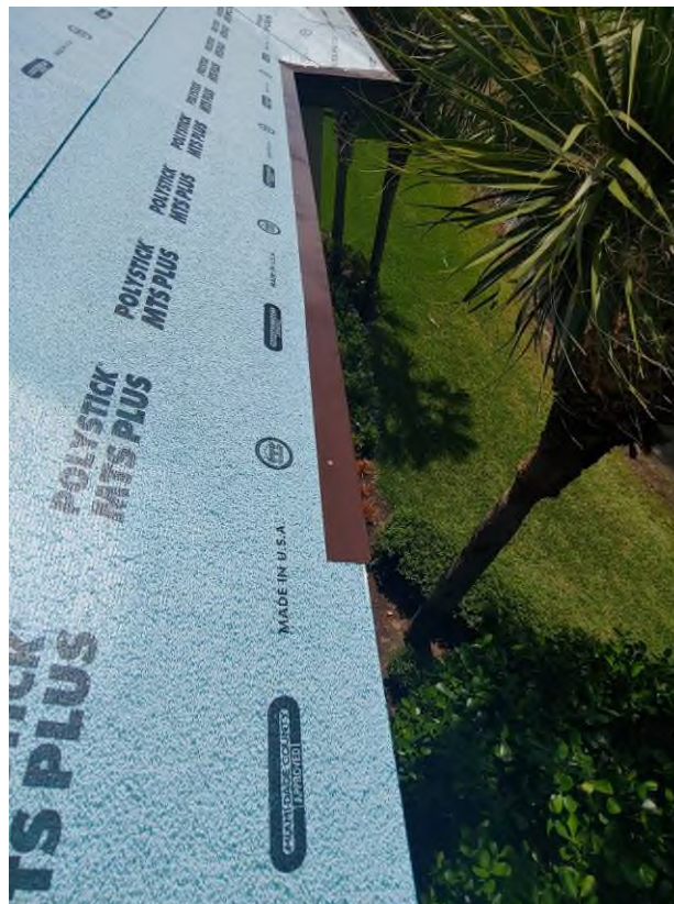
Photograph #22: Drip-edge installation was in progress on building 21810.
