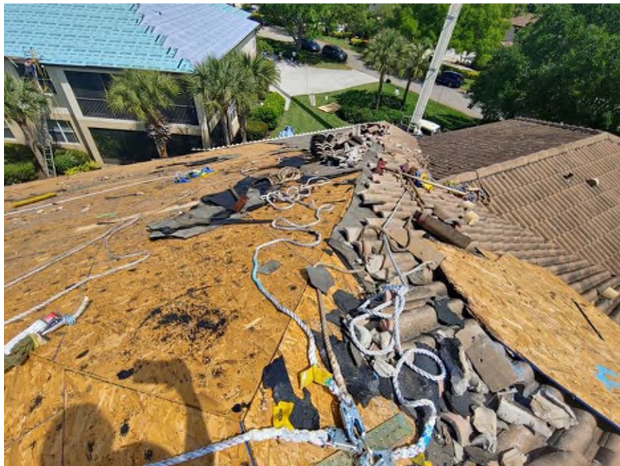
Photograph #12: Roof tile removal was in progress on 21810.
