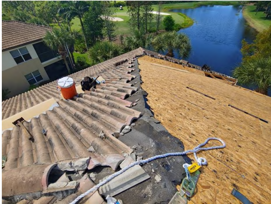
Photograph #11: Roof tile removal was in progress on 21810.
