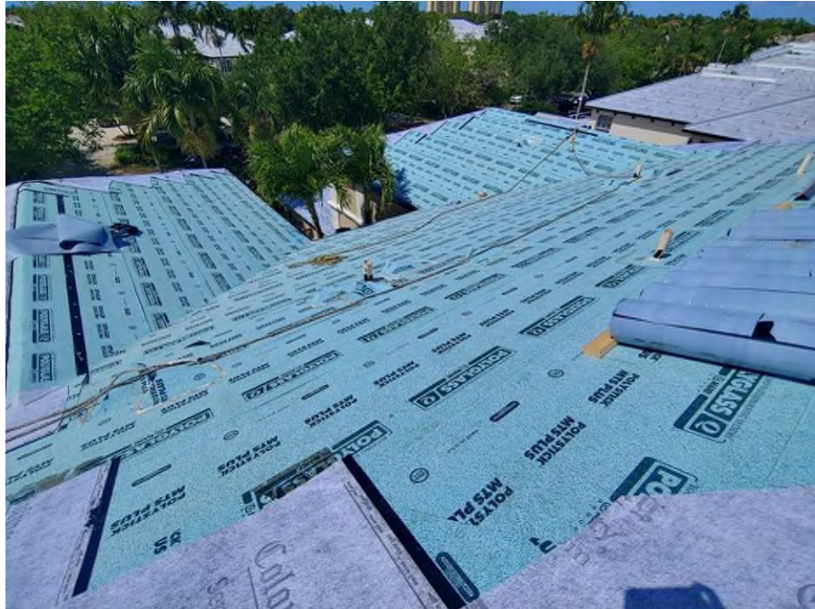
Photograph #1: Polystick MTS Plus underlayment installation was completed on building 21761.
