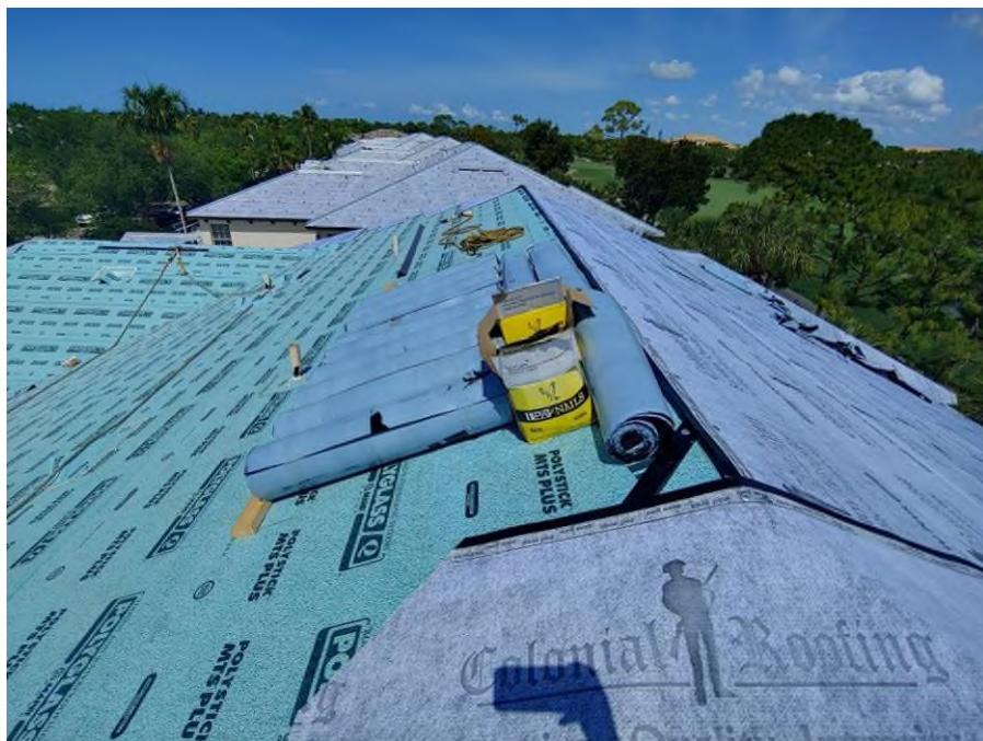
Photograph #2: Polystick MTS Plus underlayment installation was completed on building 21761.
