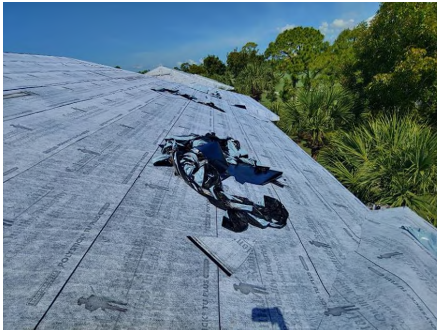
Photograph #3: Second layer of underlayment installation was in progress on building 21761.
