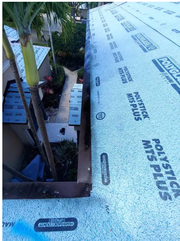
Photograph #6: Drip-edge installation was completed on the main roof of building 21761.
