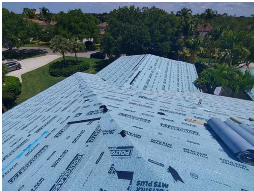
Photograph #20: Polystick MTS Plus underlayment was completed on building 21810.
