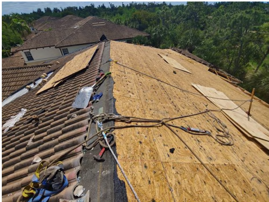
Photograph #26: Roof tile removal was in progress on building 21820.
