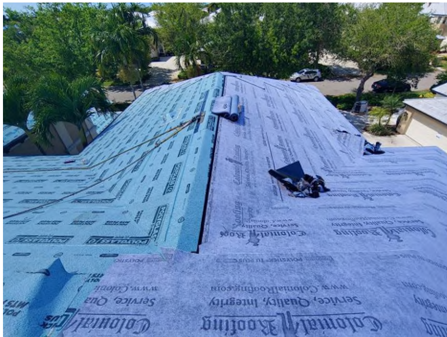
Photograph #4: Second layer of underlayment installation was in progress on building 21761.
