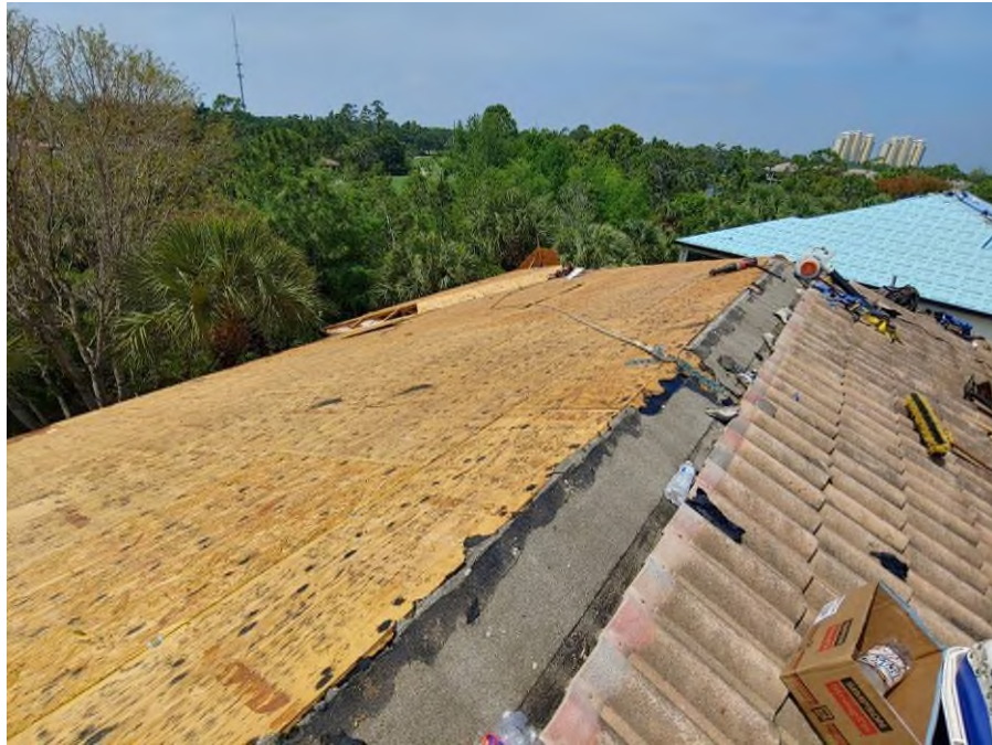
Photograph #5: Roof tile removal was in progress on building 21850.
