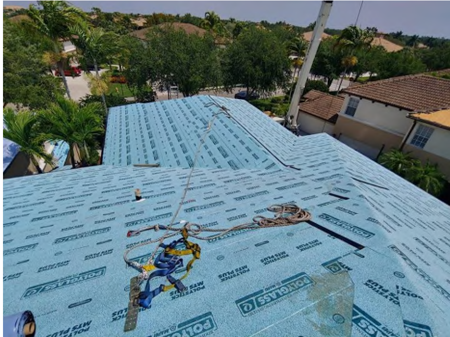
Photograph #1: Polystick MTS Plus underlayment installation was completed on building 21840.
