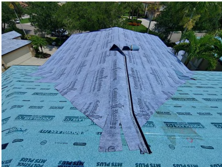
Photograph #2: Second layer of underlayment installation began on building 21840.
