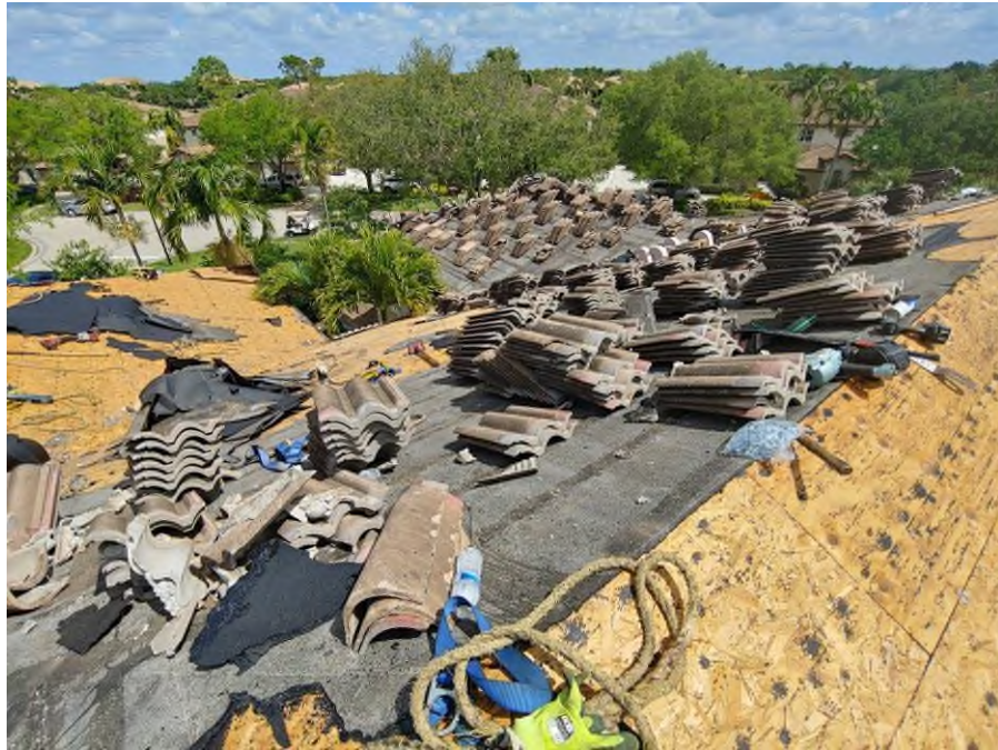
Photograph #11: Roof tile removal was in progress on building 21800.
