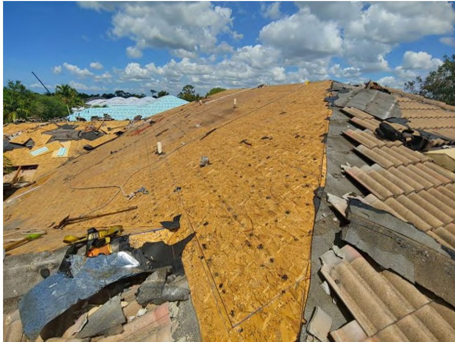
Photograph #9: Roof tile removal was in progress on building 21771.
