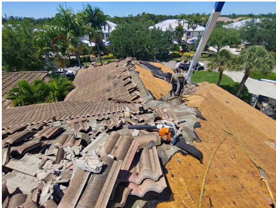
Photograph #4: Roof tile removal was in progress on building 21831.
