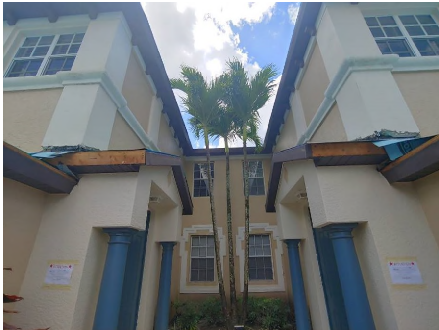
Photograph #14: Fascia repair was in progress on building 21800.
