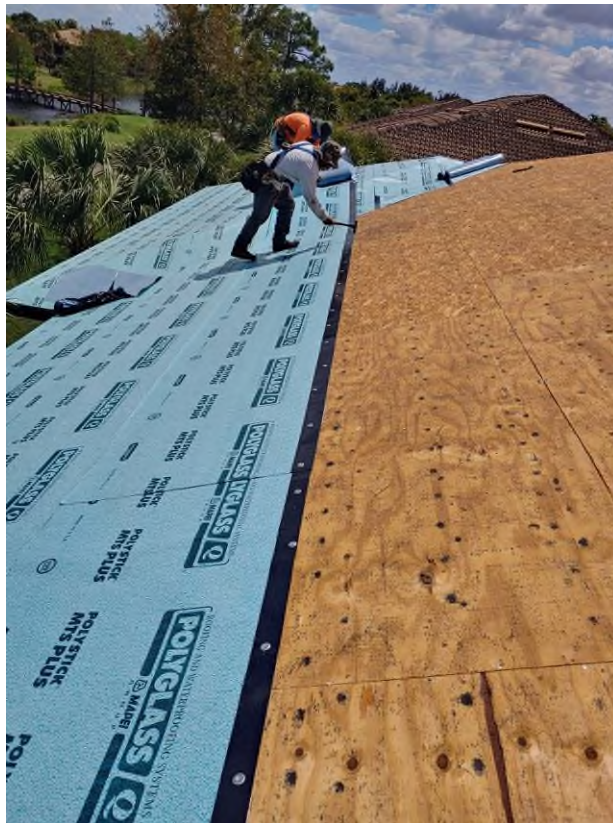
Photograph #10: Polystick MTS Plus underlayment installation was in progress on building 21761.
