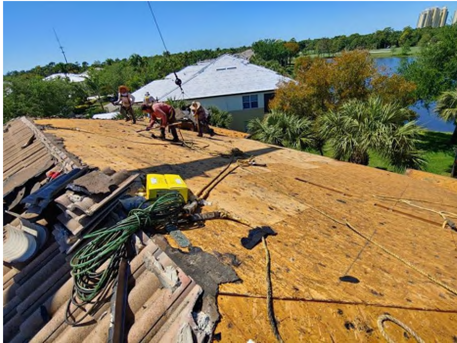
Photograph #7: Roof tile removal was in progress on building 21780.
