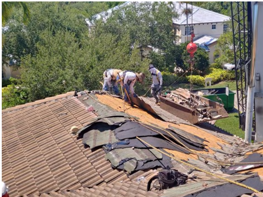
Photograph #10: Roof tile removal was in progress on building 21841.
