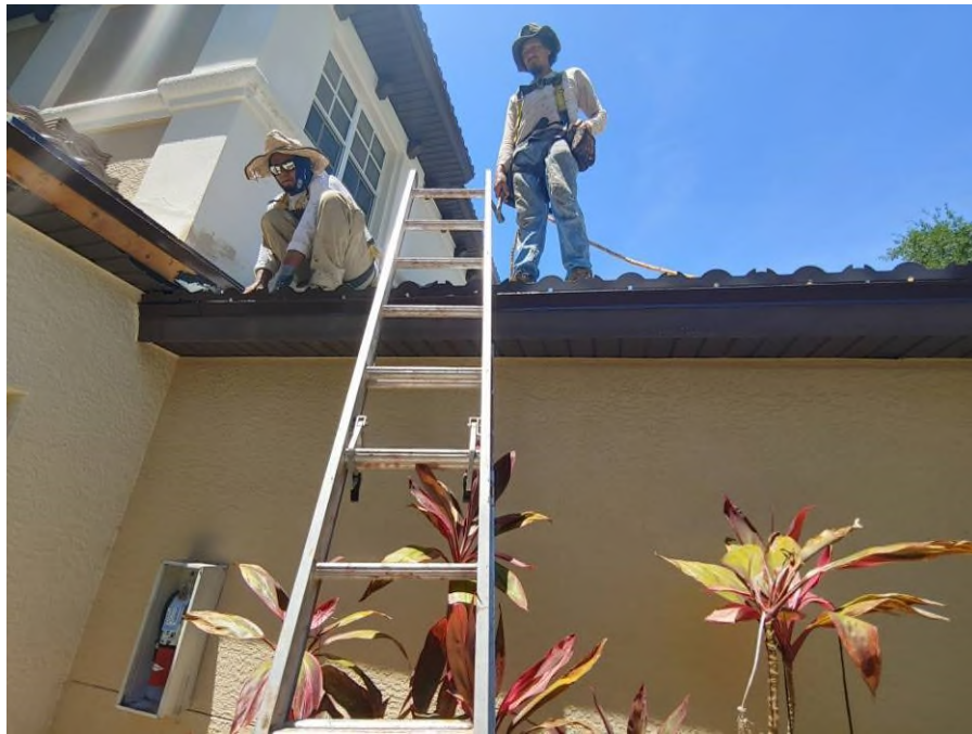
Photograph #1: Bird-stop metal flashing installation was in progress on building 21800.
