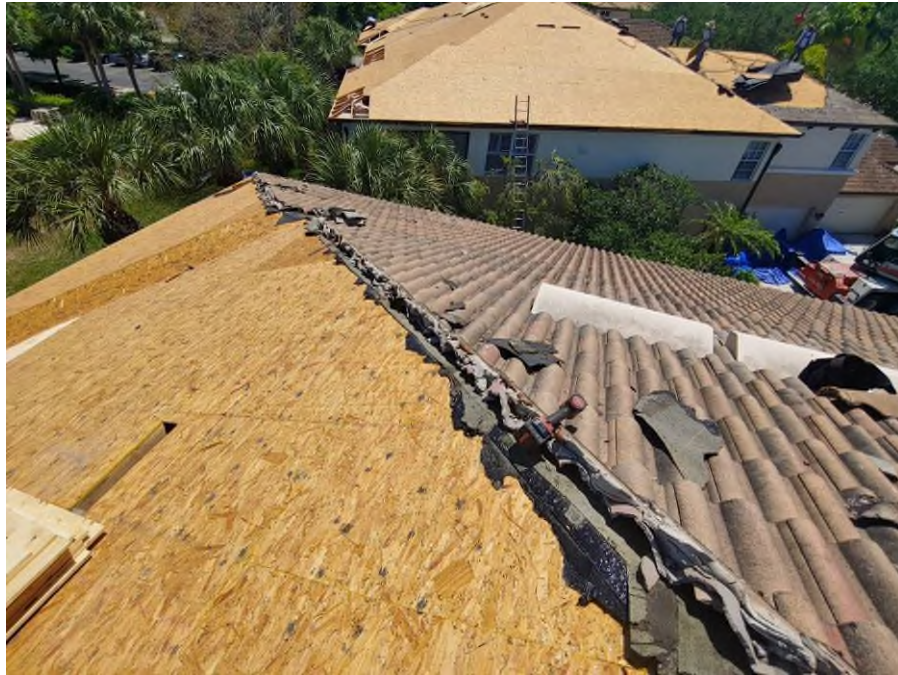
Photograph #5: Roof tile removal was in progress on building 21831.
