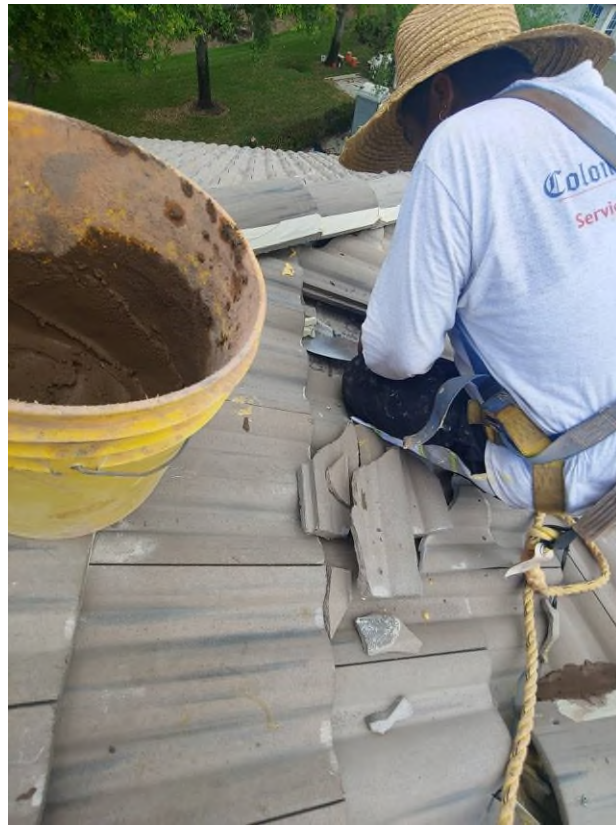
Photograph #7: Broken field tile replacement was in progress on building 21700.
