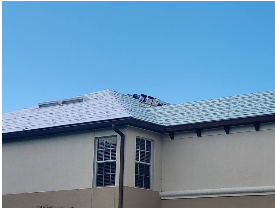
Photograph #15: Second layer of underlayment installation was in progress on building 21800.
