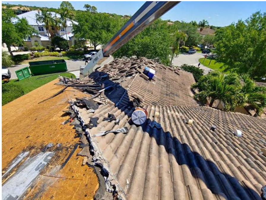
Photograph #6: Roof tile removal was in progress on building 21780.
