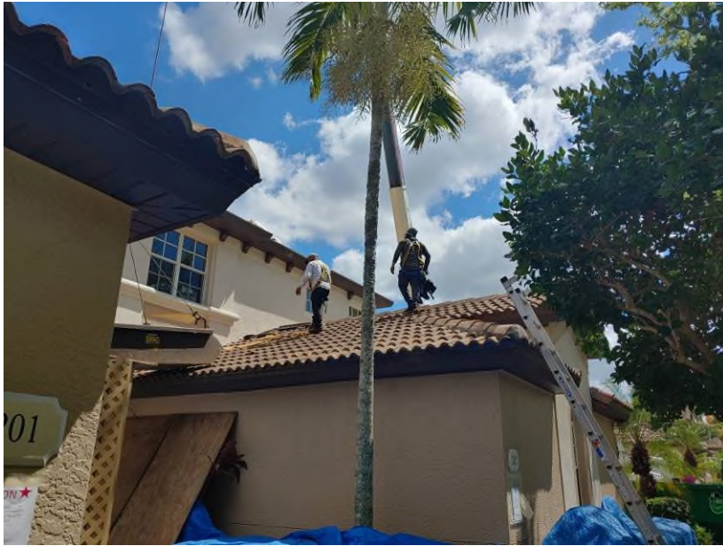
Photograph #9: Roof tile removal was in progress on on building 21761.
