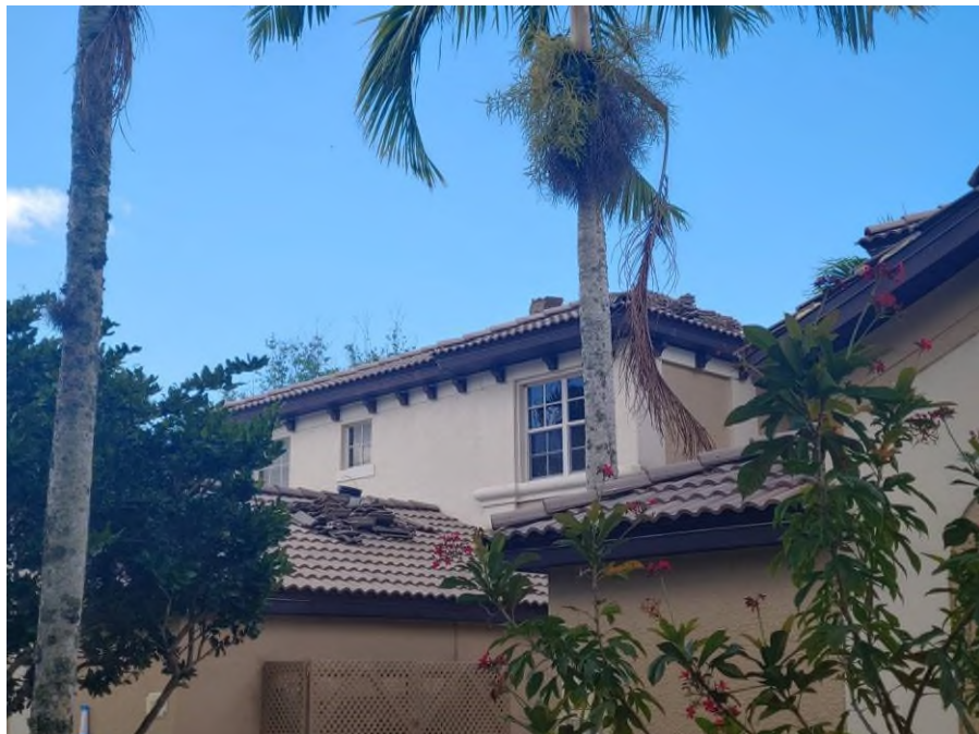
Photograph #2: Roof tile installations were in progress on building 7841.
