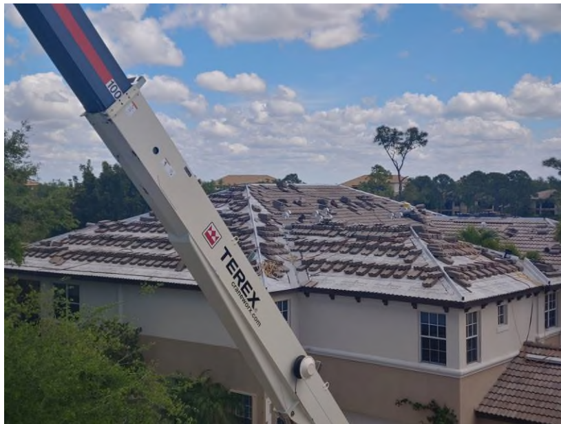
Photograph #8: Roof tiles installation were in progress on building 21711.
