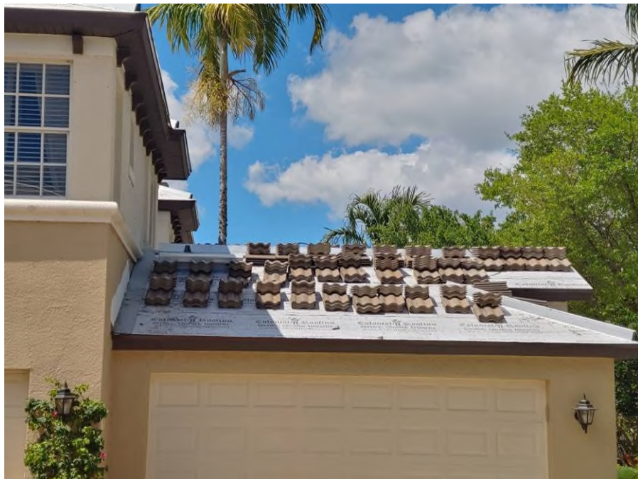
Photograph #8: Roof tiles were set in place for installation on building 21720.
