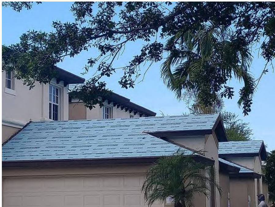
Photograph #16: Polystick MTS Plus underlayment installation was completed on building 21800.
