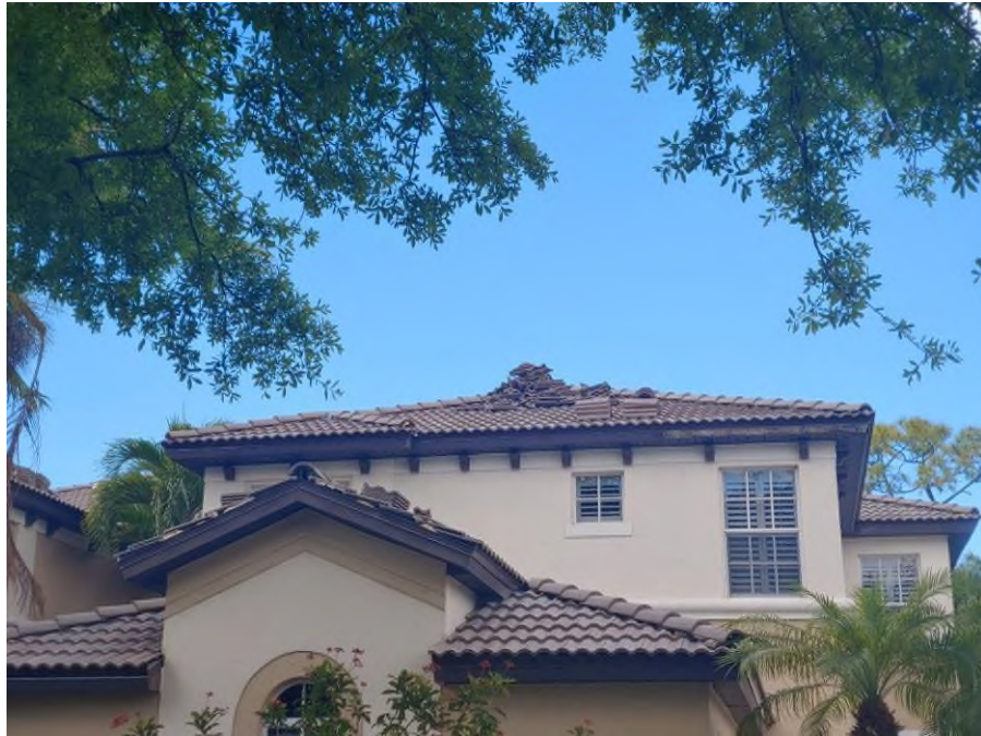
Photograph #1: Roof tile installations were in progress on building 7841.
