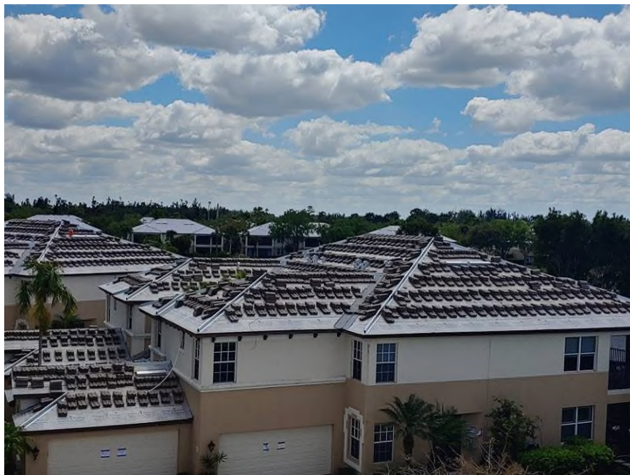
Photograph #6: Roof tiles were set in place for installation on building 21710.
