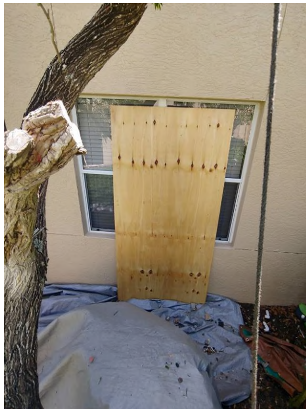
Photograph #16: Window protection installation was observed on building 21841.
