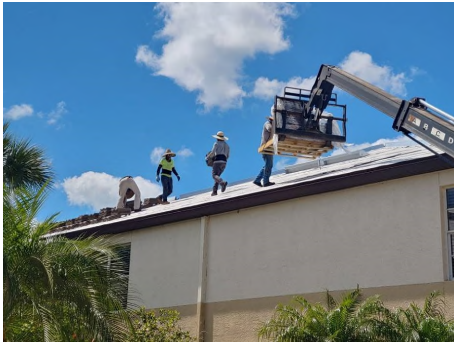
Photograph #7: Roof tiles were set in place for installation on building 21720.
