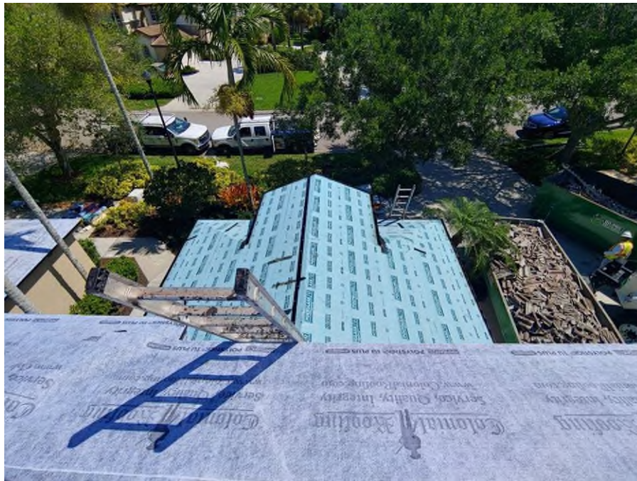
Photograph #1: Polystick MTS Plus underlayment installation was completed on building 21820.
