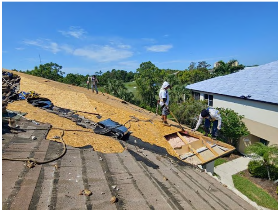
Photograph #6: Roof tile removal was in progress on building 21830.
