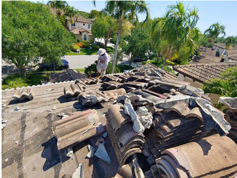
Photograph #7: Roof tile removal was in progress on building 21830.
