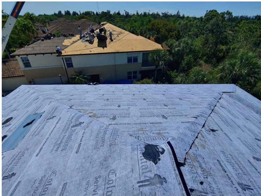
Photograph #2: Second layer of underlayment was in progress on building 21820.
