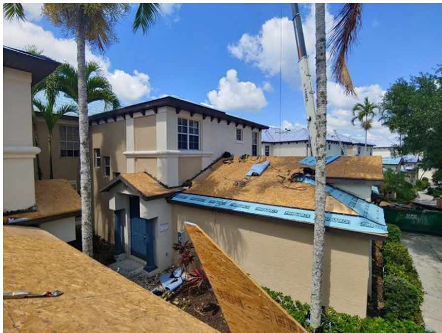
Photograph #10: Polystick MTS Plus underlayment installation was in progress on building 21830.
