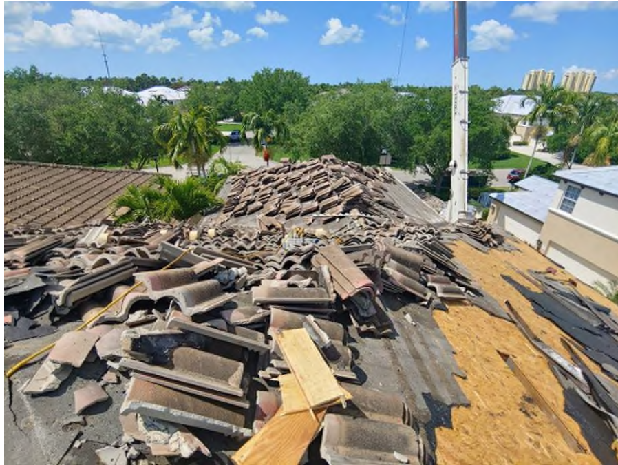
Photograph #1: Roof tile removal was in progress on building 21791.
