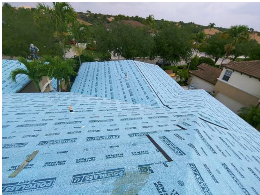
Photograph #4: Polystick MTS Plus underlayment installation was completed on building 21840.
