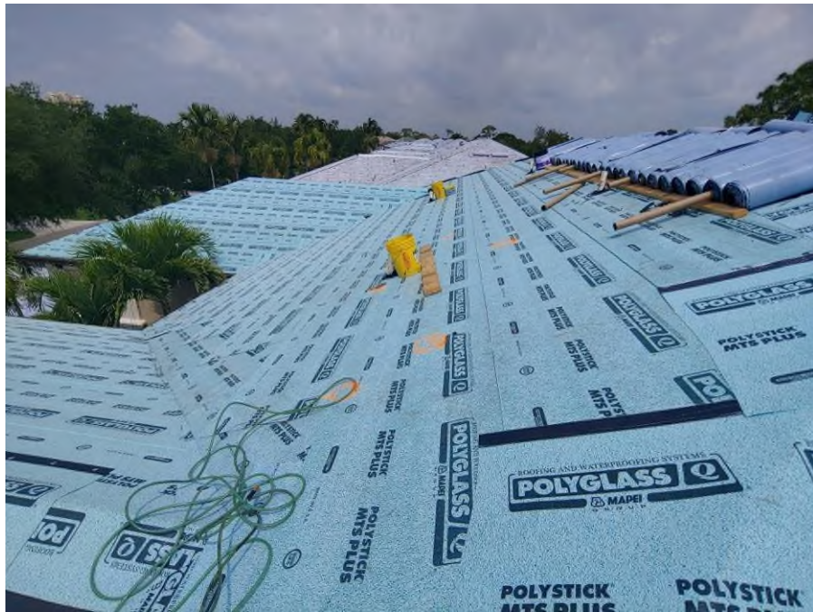
Photograph #1: Polystick MTS Plus underlayment installation was completed on building 21791.
