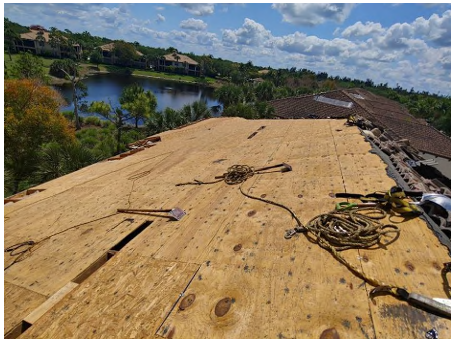
Photograph #2: Roof tile removal was in progress on building 21791.
