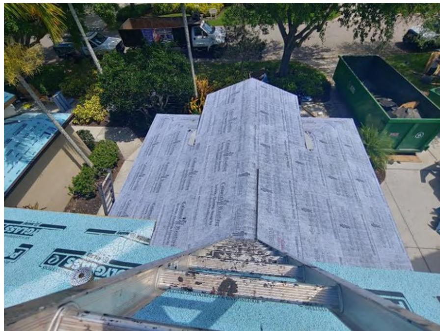
Photograph #24: Second layer of underlayment began on building 21810.
