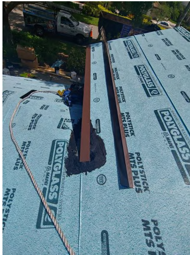
Photograph #23: Drip-edge installation was in progress on building 21810.
